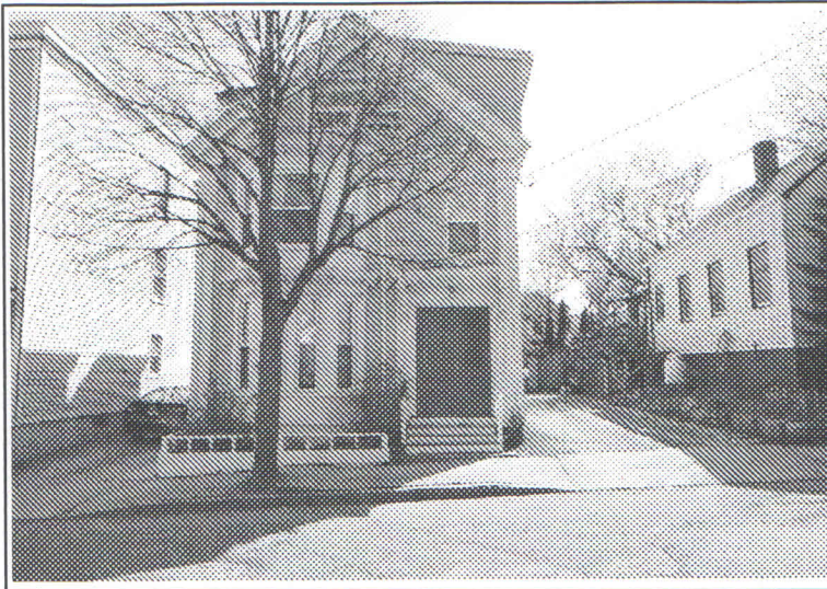
FRONT OF SUBJECT PROPERTY
