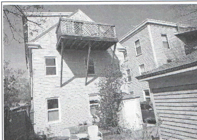
REAR OF SUBJECT PROPERTY
