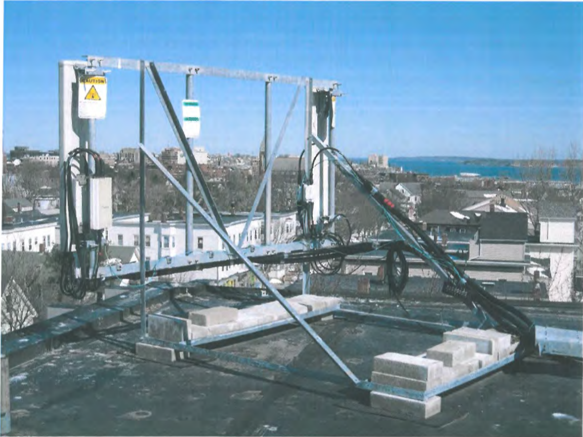
Photo 4: Sample photo illustrating the existing antenna supported on a ballast mount.
