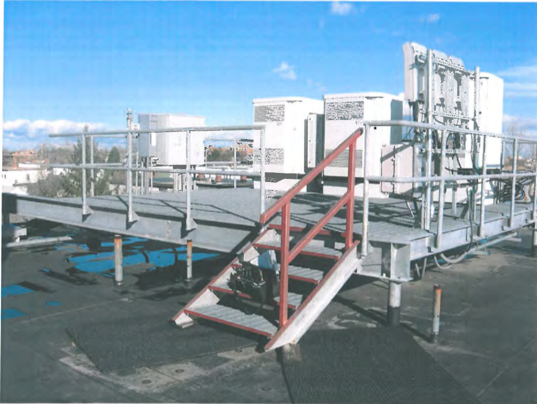
Photo 1: Sample photo illustrating the existing equipment platform
