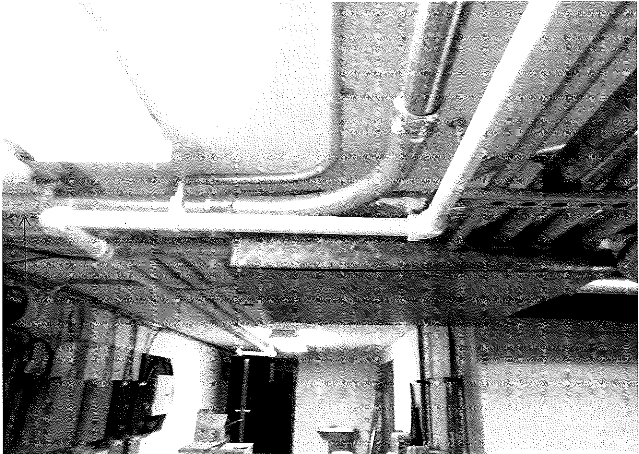
New Conduit Run to Equipment on Roof
