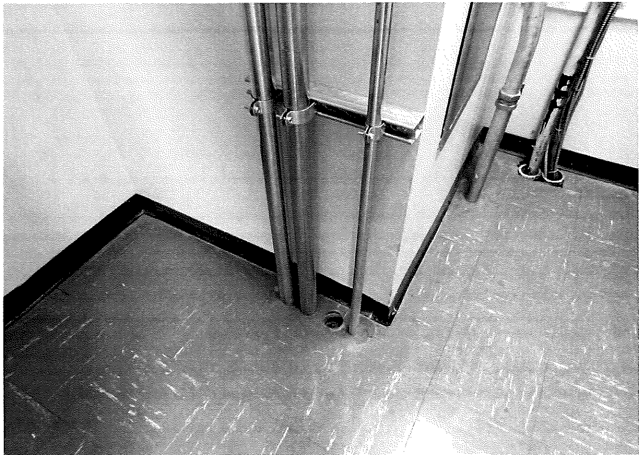
New Conduit Run (Continued)
