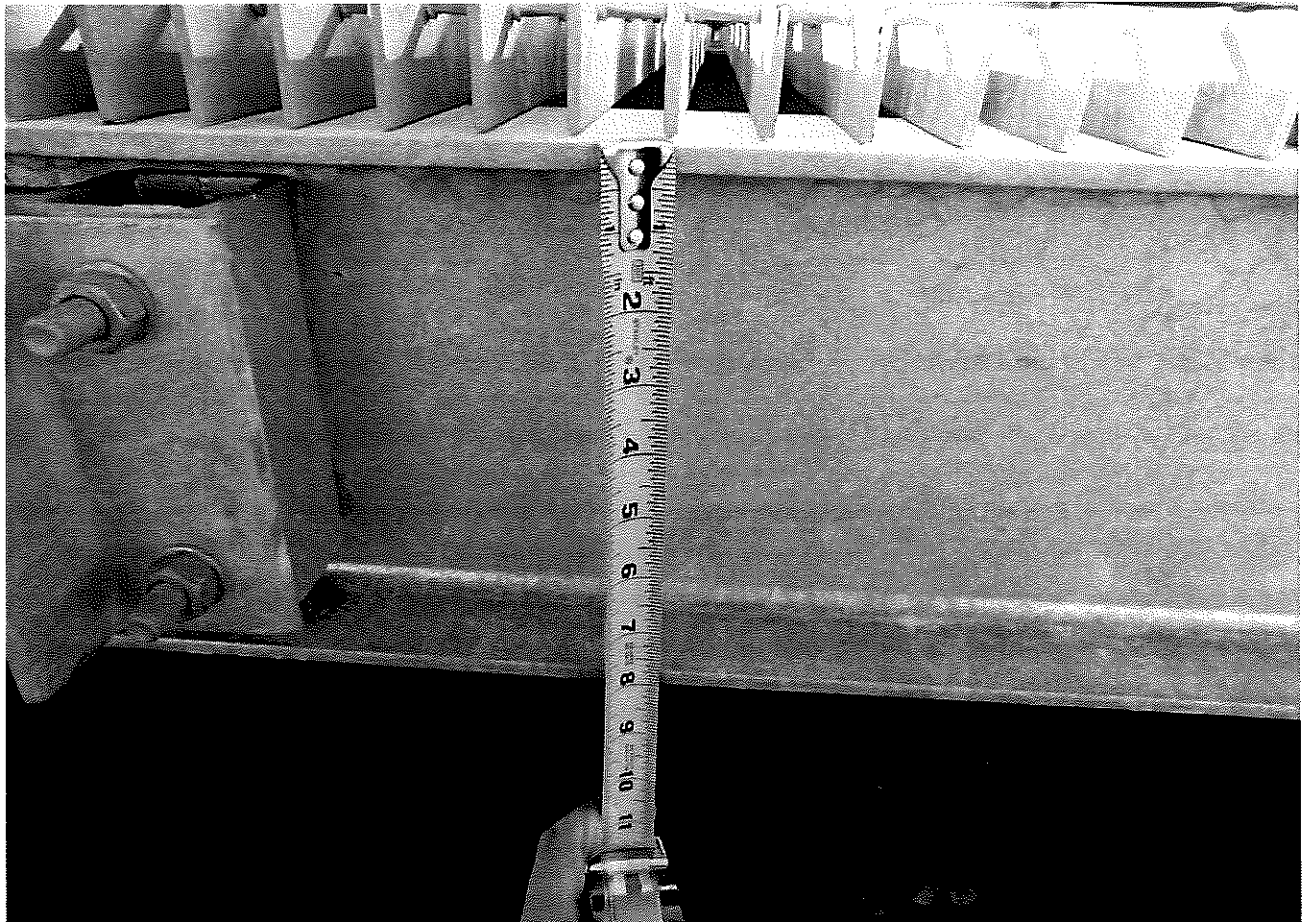
New Equipment Frame Support Beam
