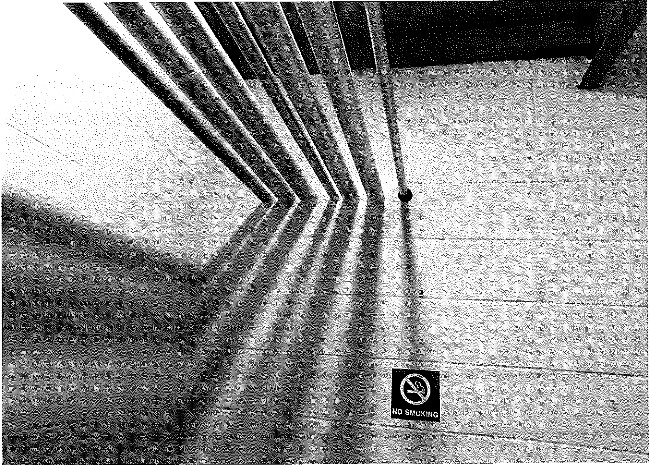
New Conduit Run (Continued)
