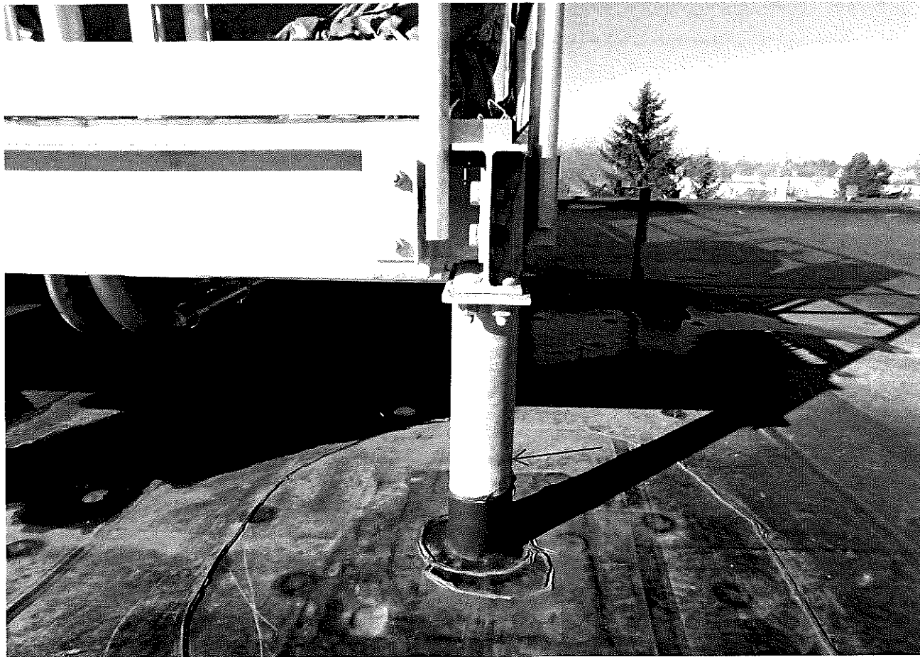
New Equipment Frame Post Downs
