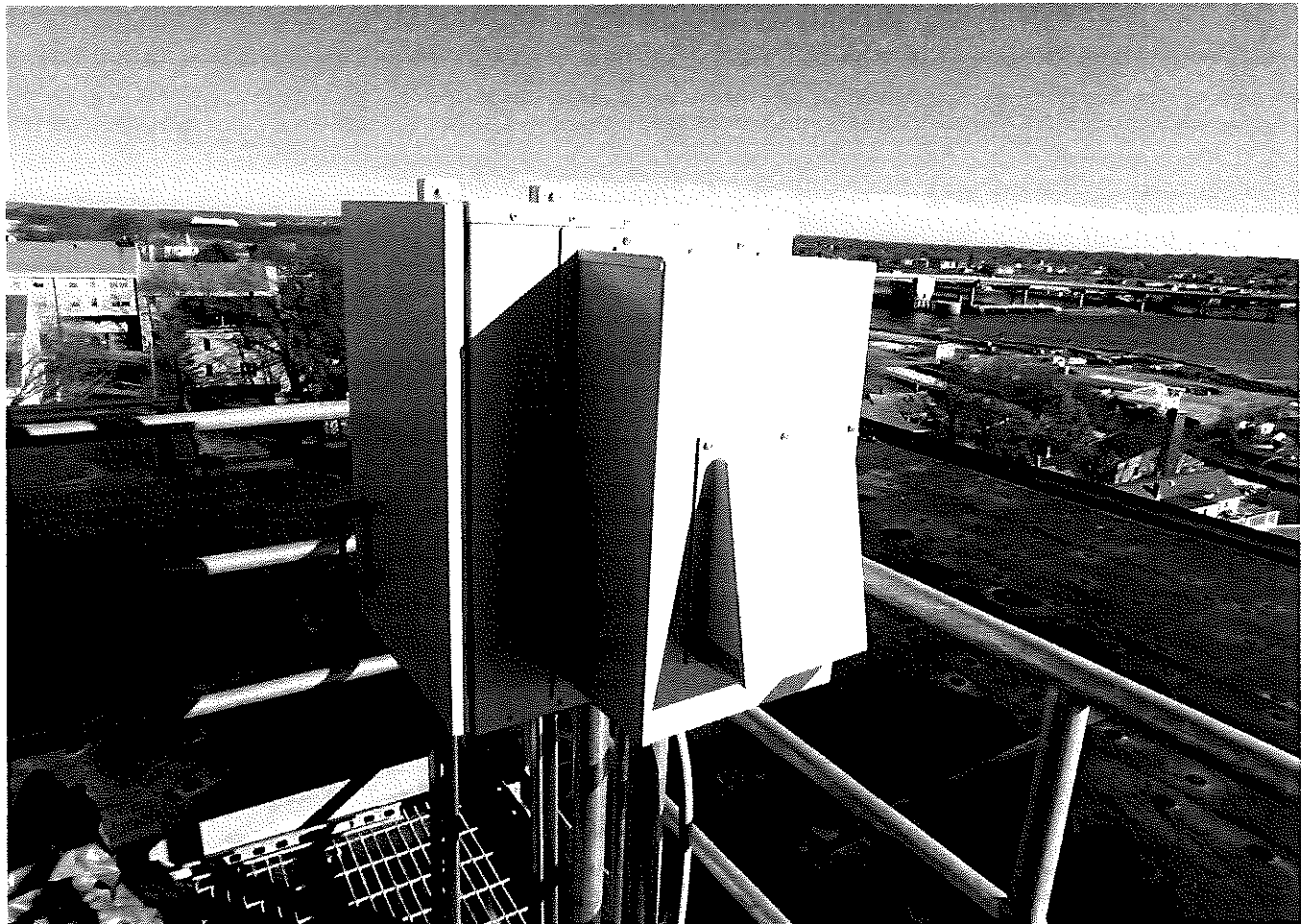
New RAC24 Cabinet
