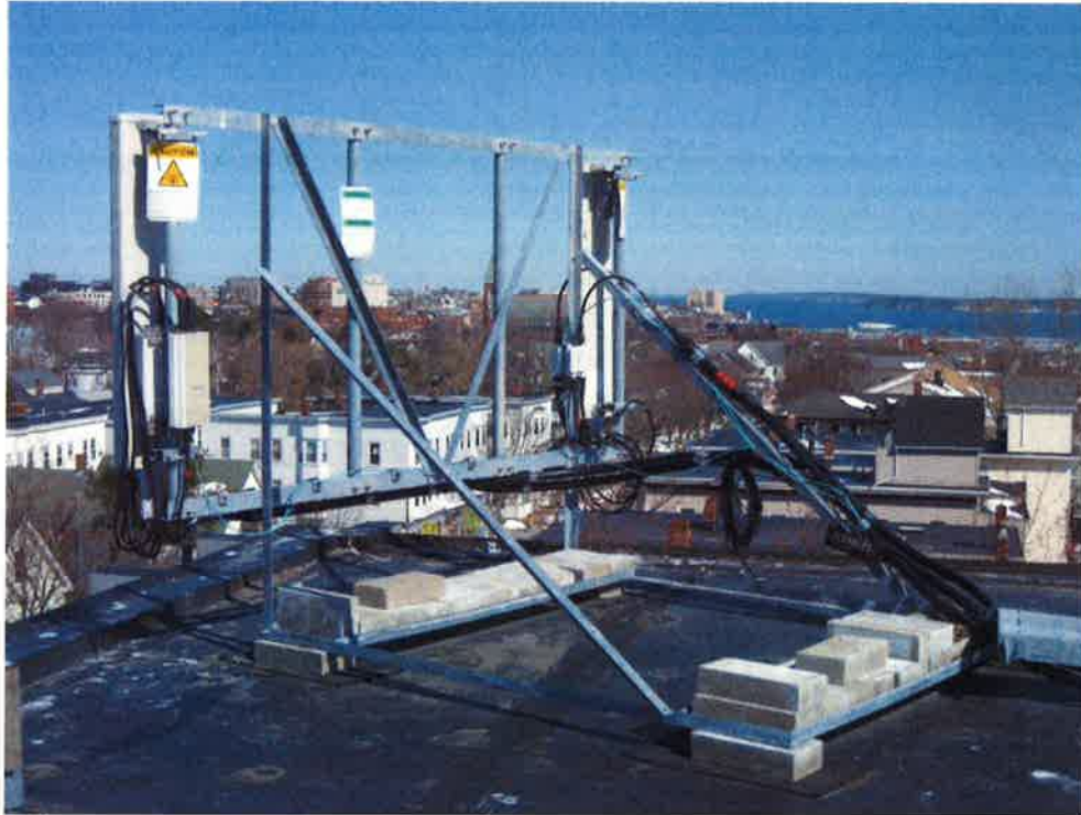
Photo 1: Sample photo illustrating the existing non-penetrating ballast frame.
