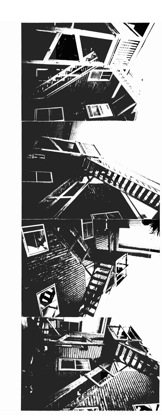
Szetional 261 DAN forth St-Brad Marrison Stair Standl SZX6PTLumber -7/11"? Ø! Stringer is Stringer is Pressure Tracted 2×12 GXTENOV STAW Or Fire Oscape. Stairs are & inch risers
