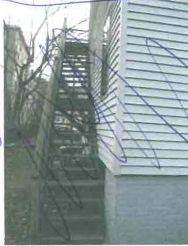
6) Rear elevation, fire escape
