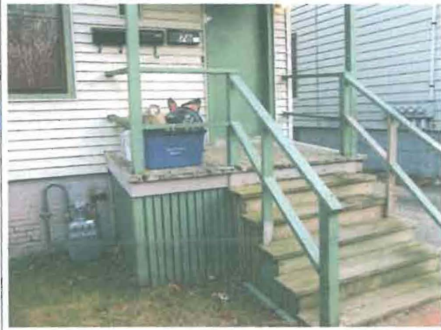
4) View of common gas meter and front entry upper floors
