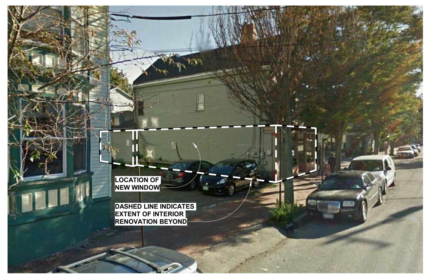
EXISTING - ALONG PINE STREET APPROACHED FROM BRACKETT STREET
