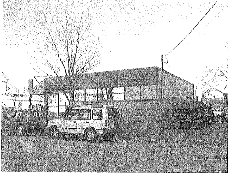
Front and side view from Pine Street.
