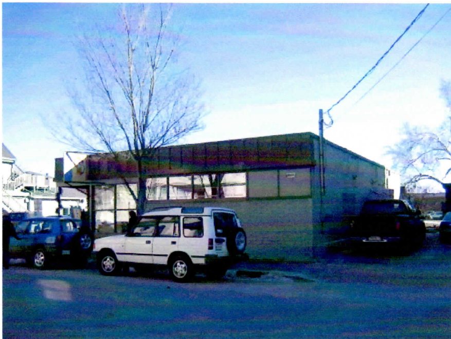
Front and side view from Pine Street.
