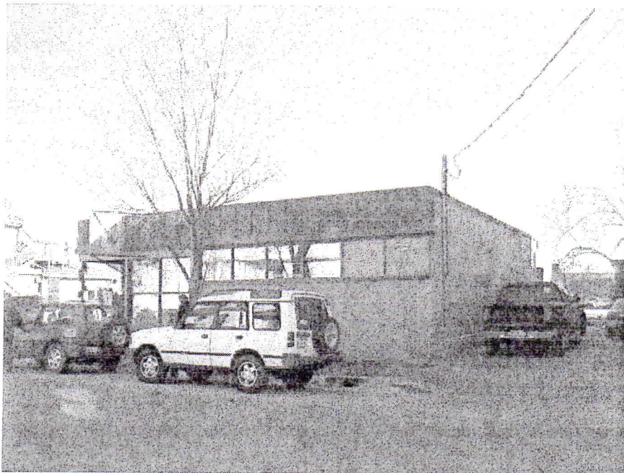
Front and side view from Pine Street.
