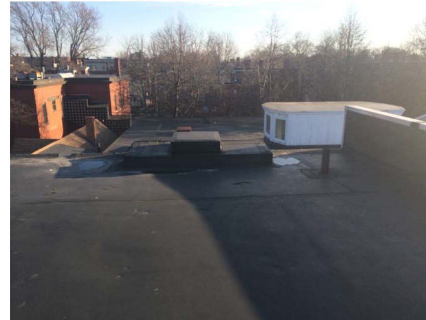
EXISTING CONDITION | LOOKING TOWARDS EXISTING HATCH
