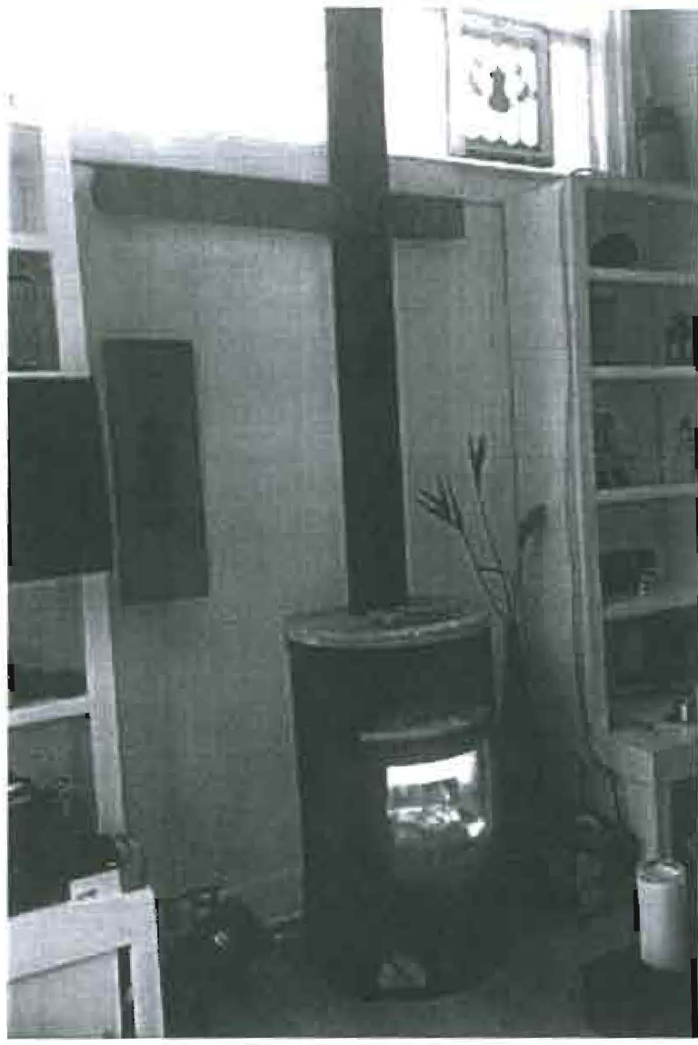
(Stove is installed on a glass hearth pad).
