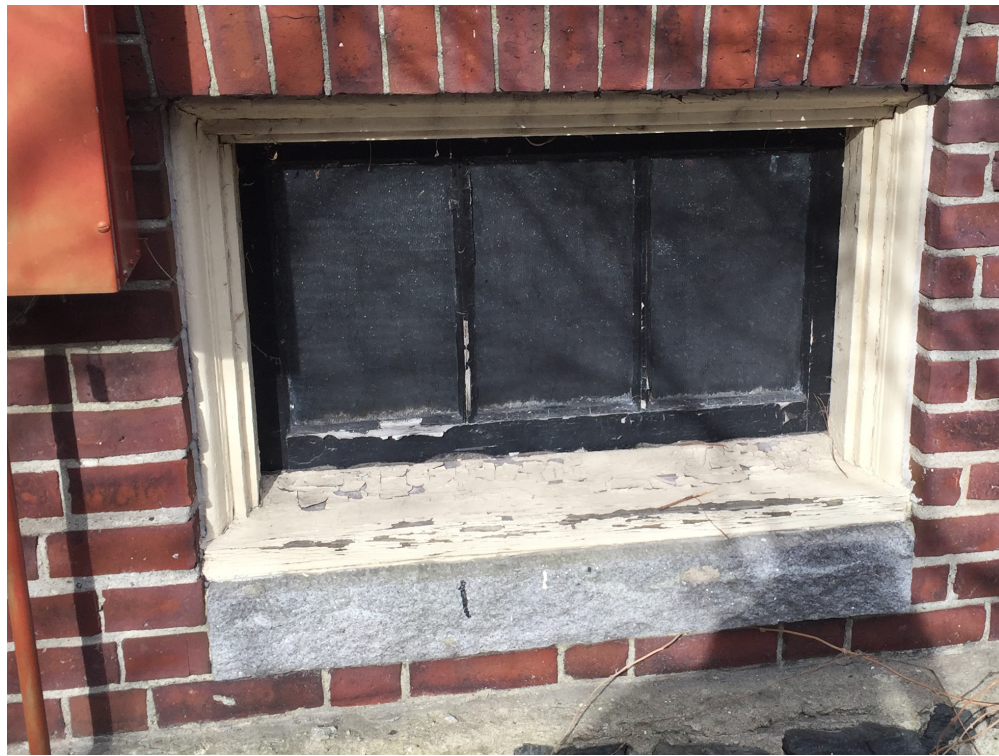
EXISTING BASEMENT WINDOW
