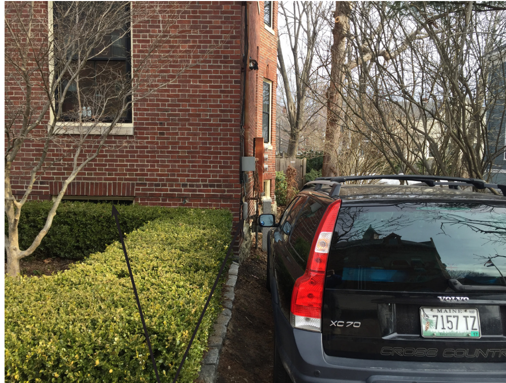
DRIVEWAY VIEW, SHOWS (2) WDOS NOT TO BE REPLACED
