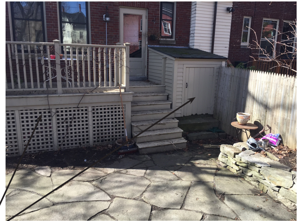
BACKYARD NOT VISIBLE FROM ANY STREET OR PUBLIC VIEWING POINT. REAR WINDOW UNDER EXISTING DECK. DOOR OPENING TO BE ENLARGED DOWN, EXISTING HEADER TO BE RETAINED
