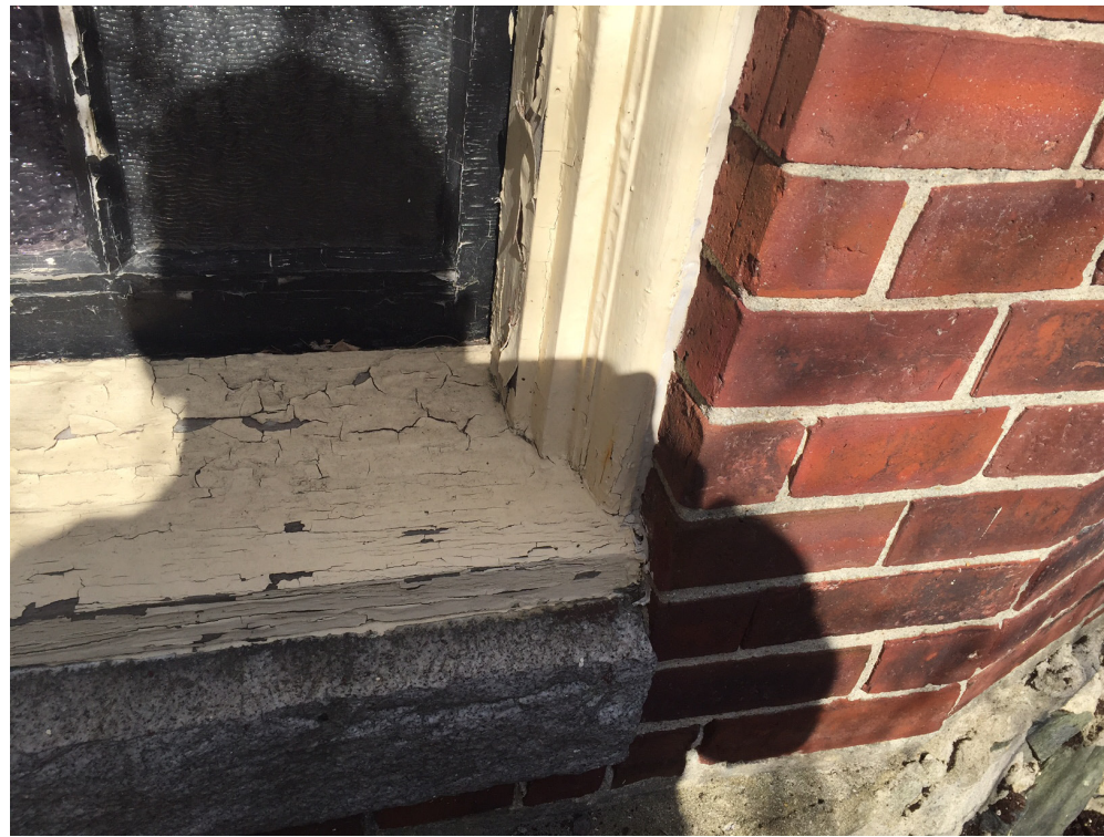
EXISTING BASEMENT WINDOW
