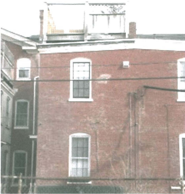
Existing sun deck at 91 Pine, viewed from the rear alleyway.
