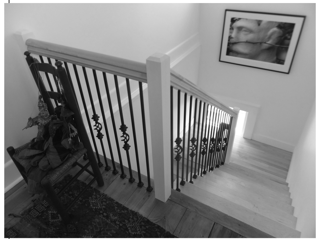
EXISTING RAILING SIMILAR TO NEW
