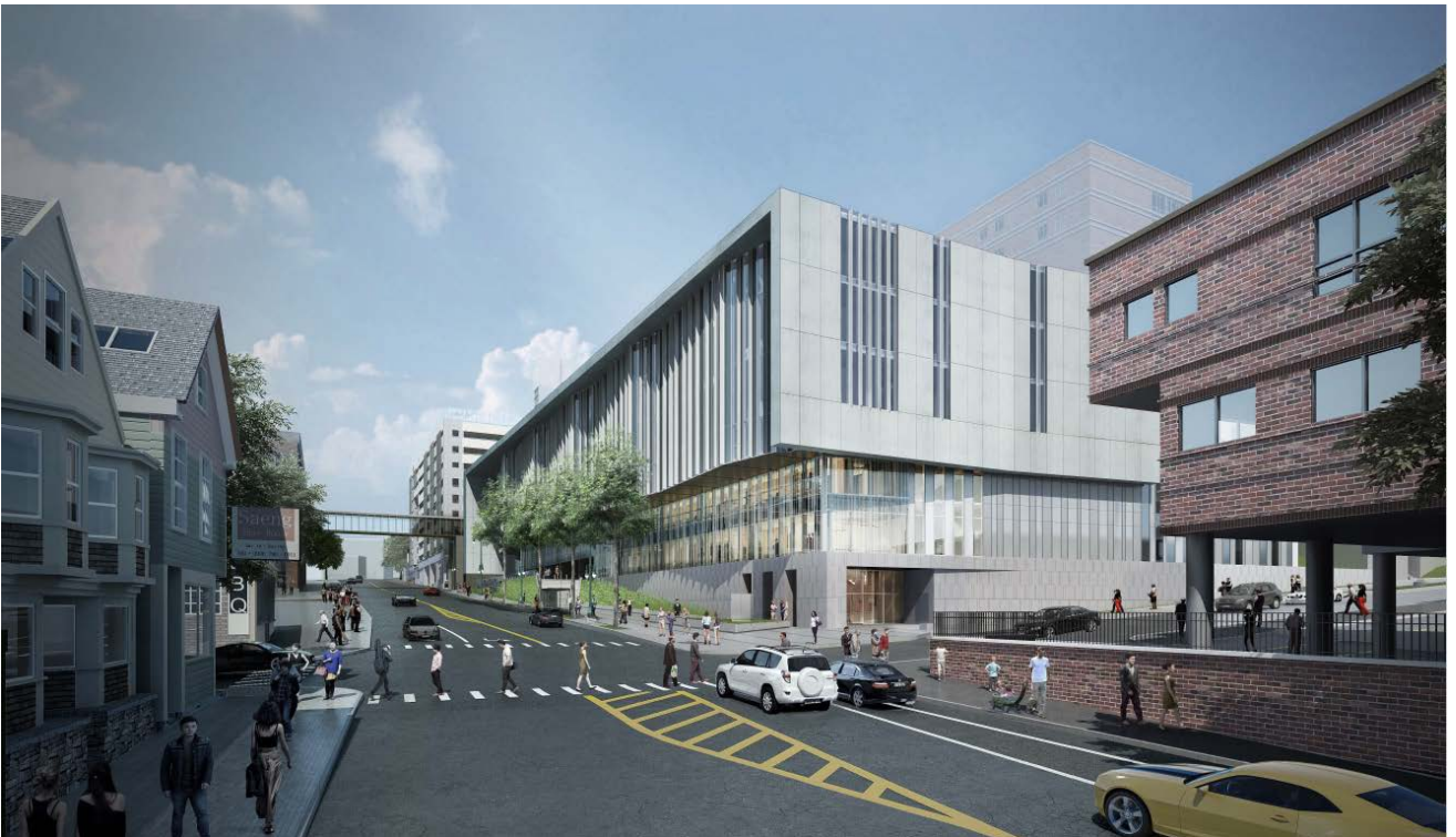
Figures 7 and 8: View from Congress Street looking east, existing (above) and proposed (below)
