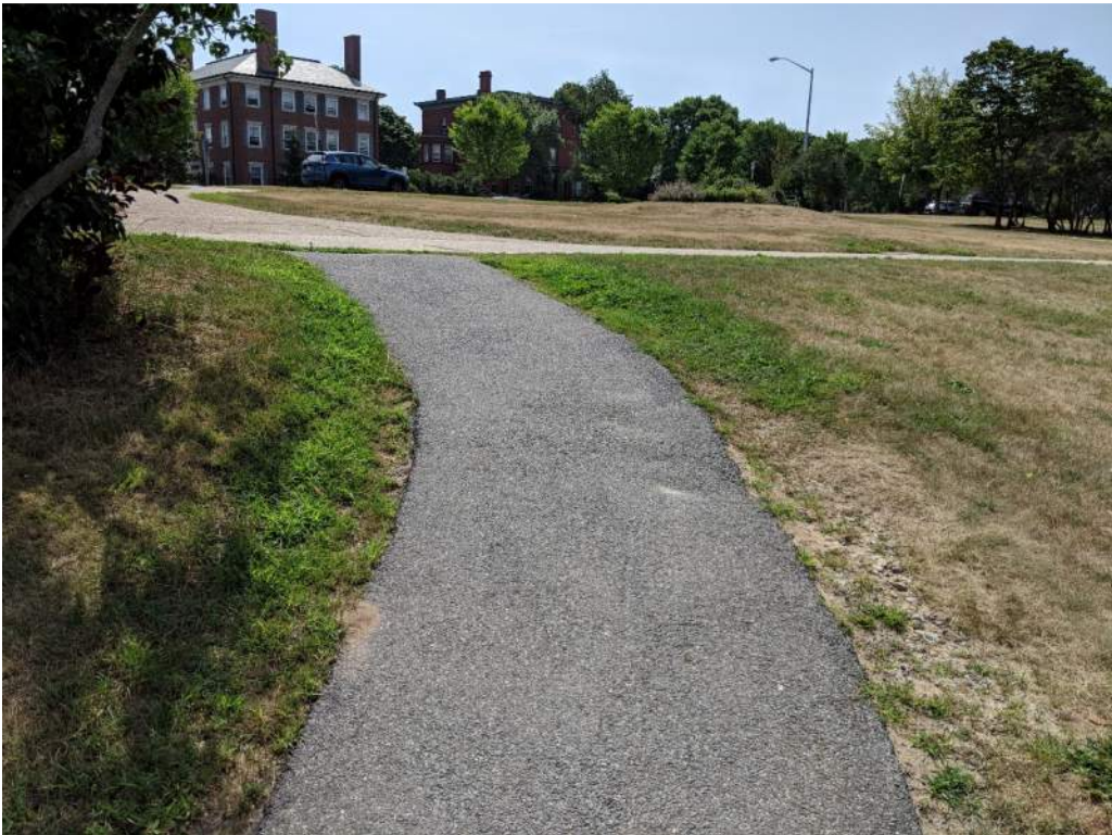
Photo 14: Trail section in good condition
