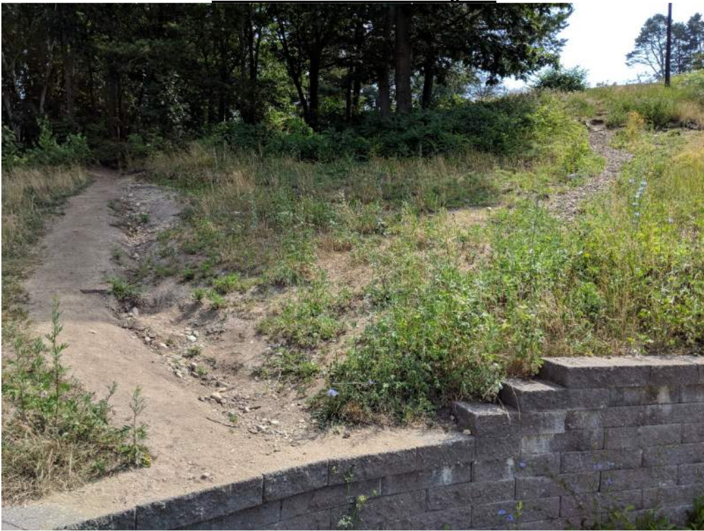
Photo 2: Foot path connection at top of retaining wall
