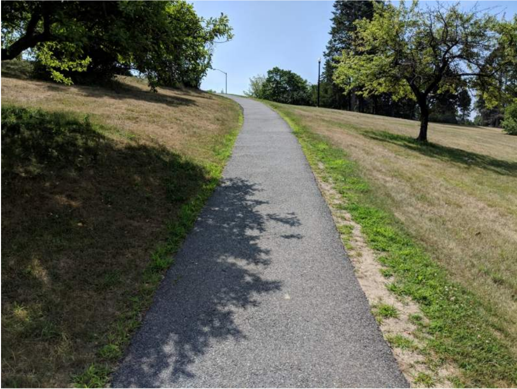
Photo 13: Trail section in good condition
