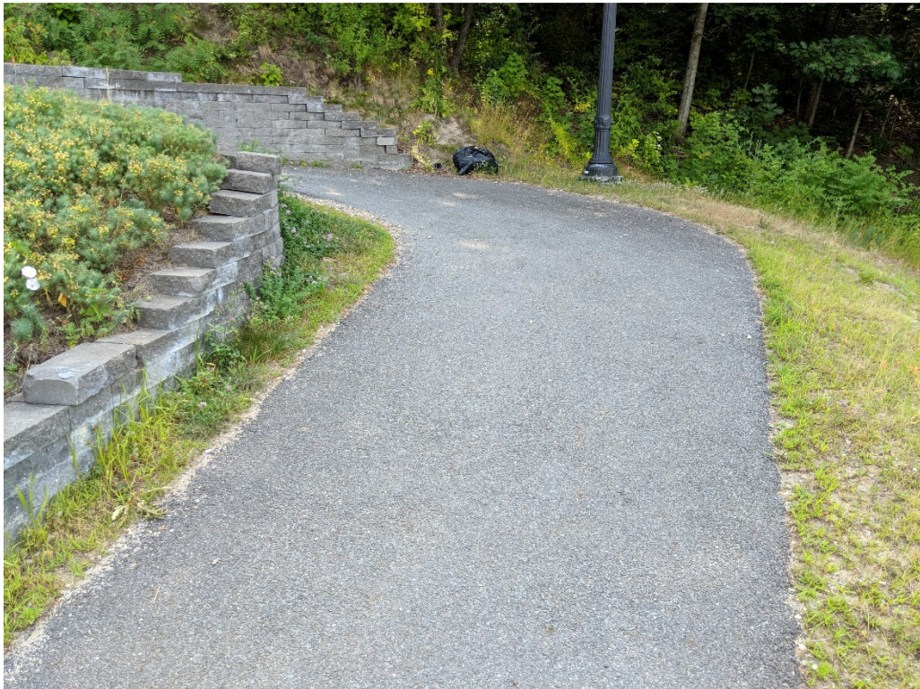
Photo 4: Trail section in good condition
