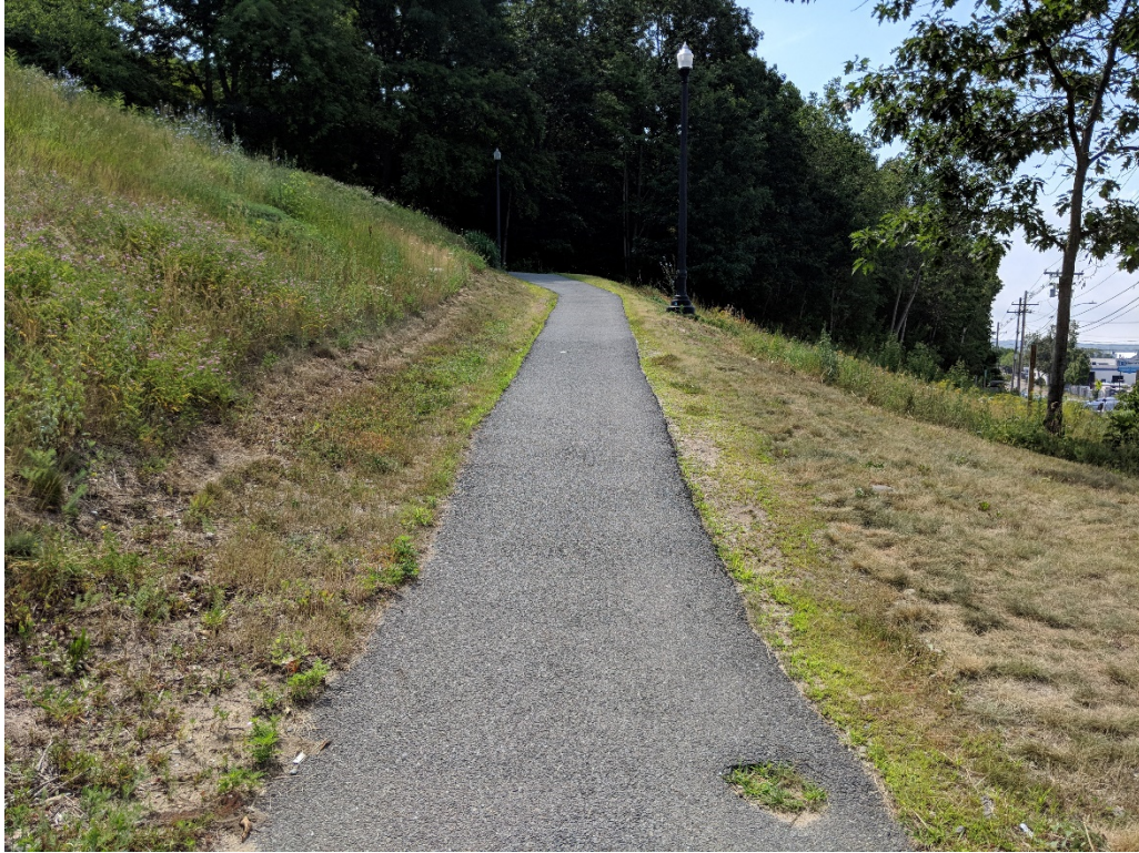
Photo 3: Trail section in good condition
