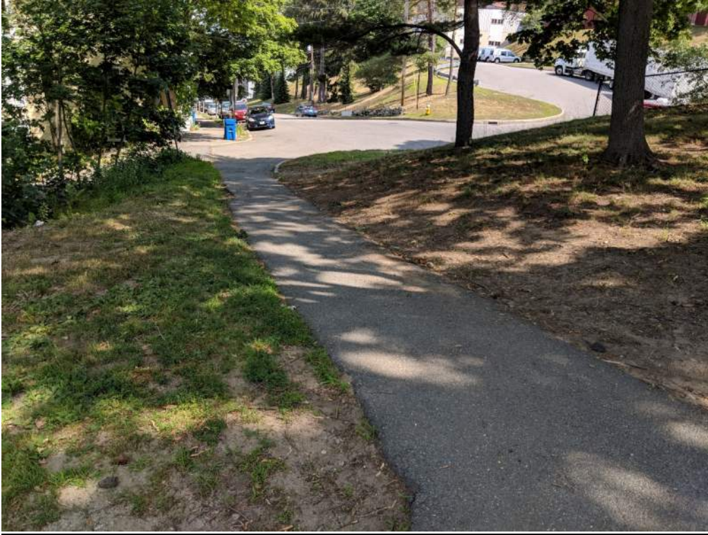
Photo 11: Trail section in good condition
