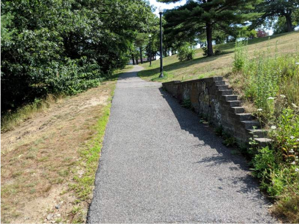
Photo 7: Trail section in good condition
