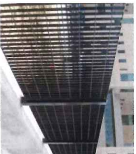
Ground Floor Security Grilles
