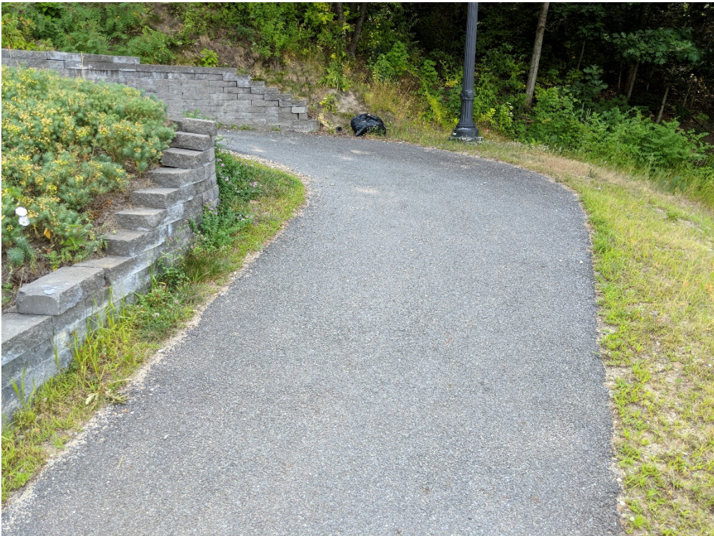
Photo 4: Trail section in good condition
