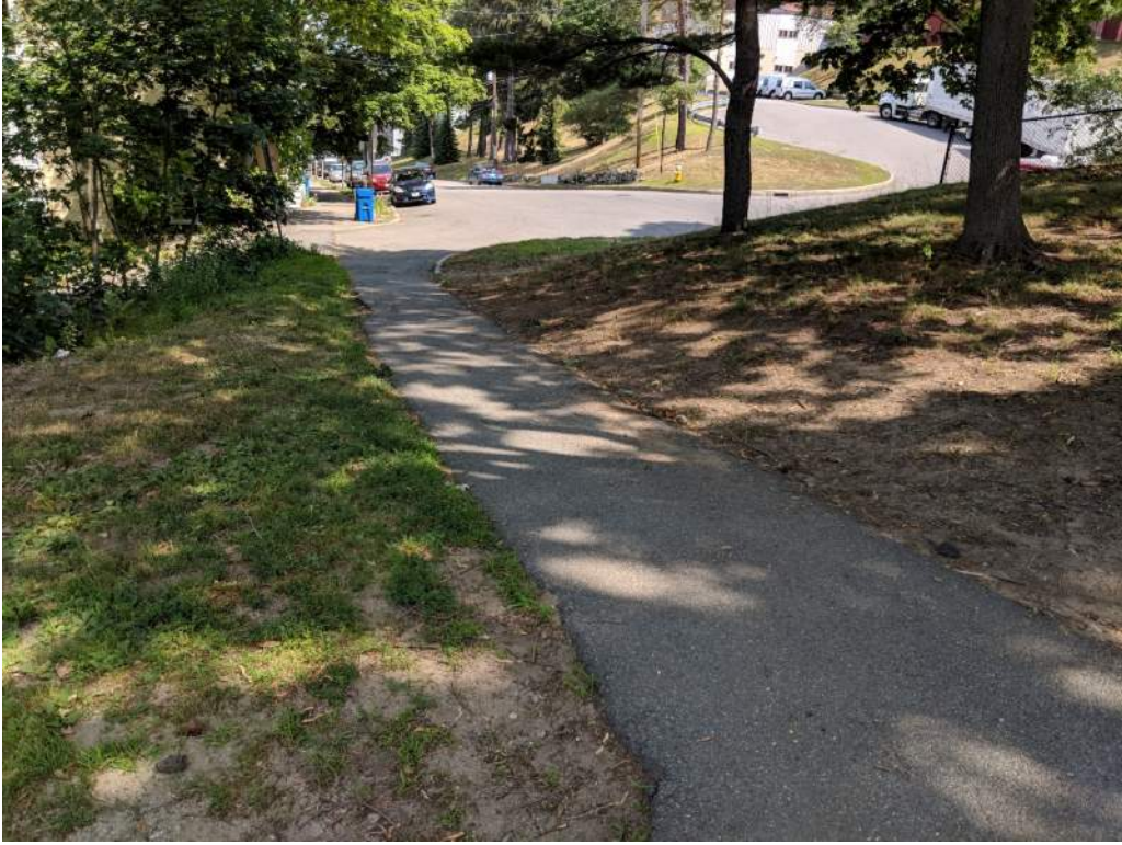
Photo 11: Trail section in good condition
