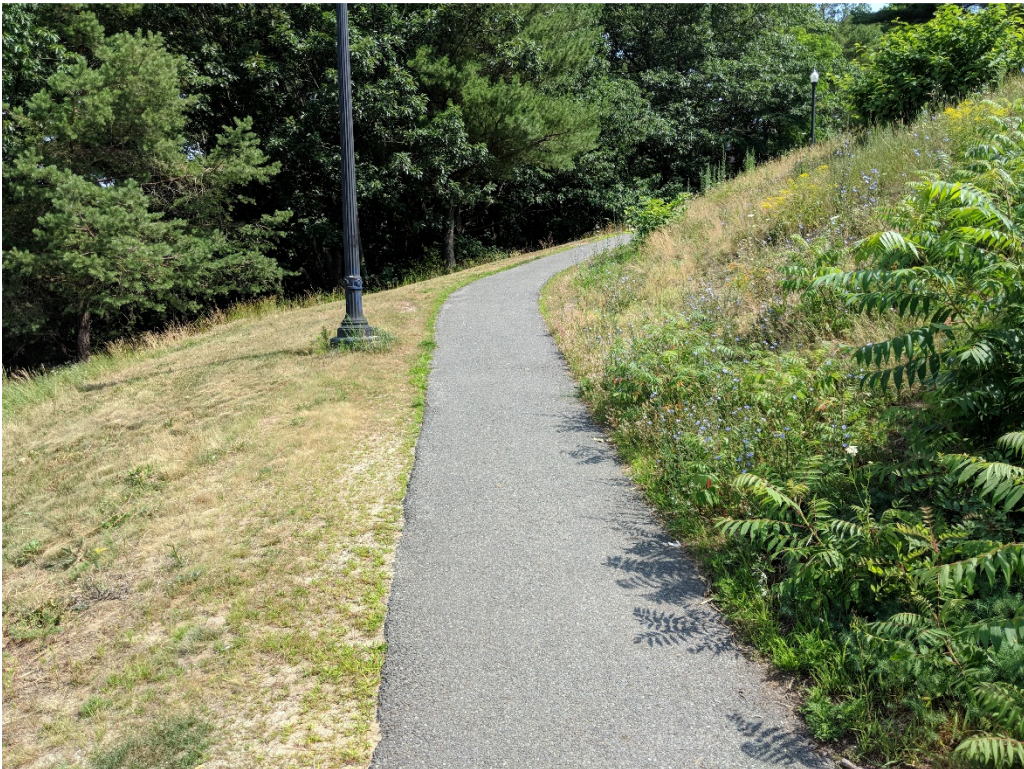
Photo 6: Trail section in good condition
