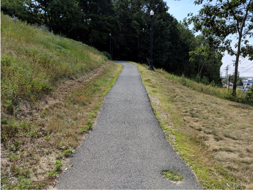
Photo 3: Trail section in good condition
