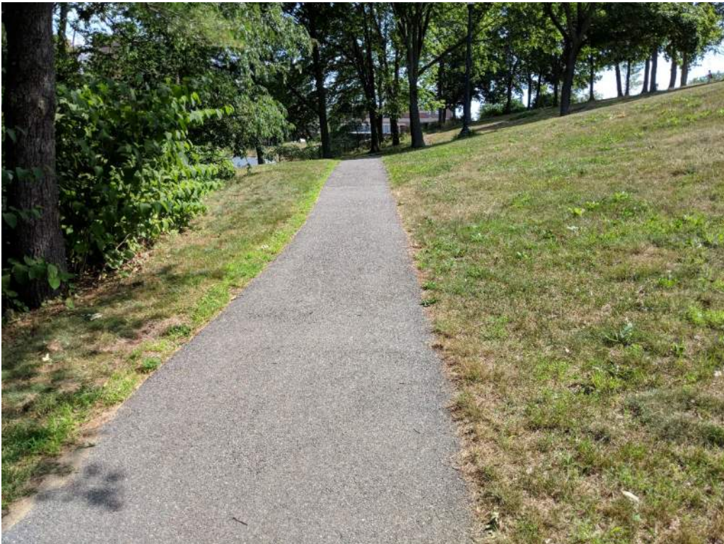
Photo 10: Trail section in good condition
