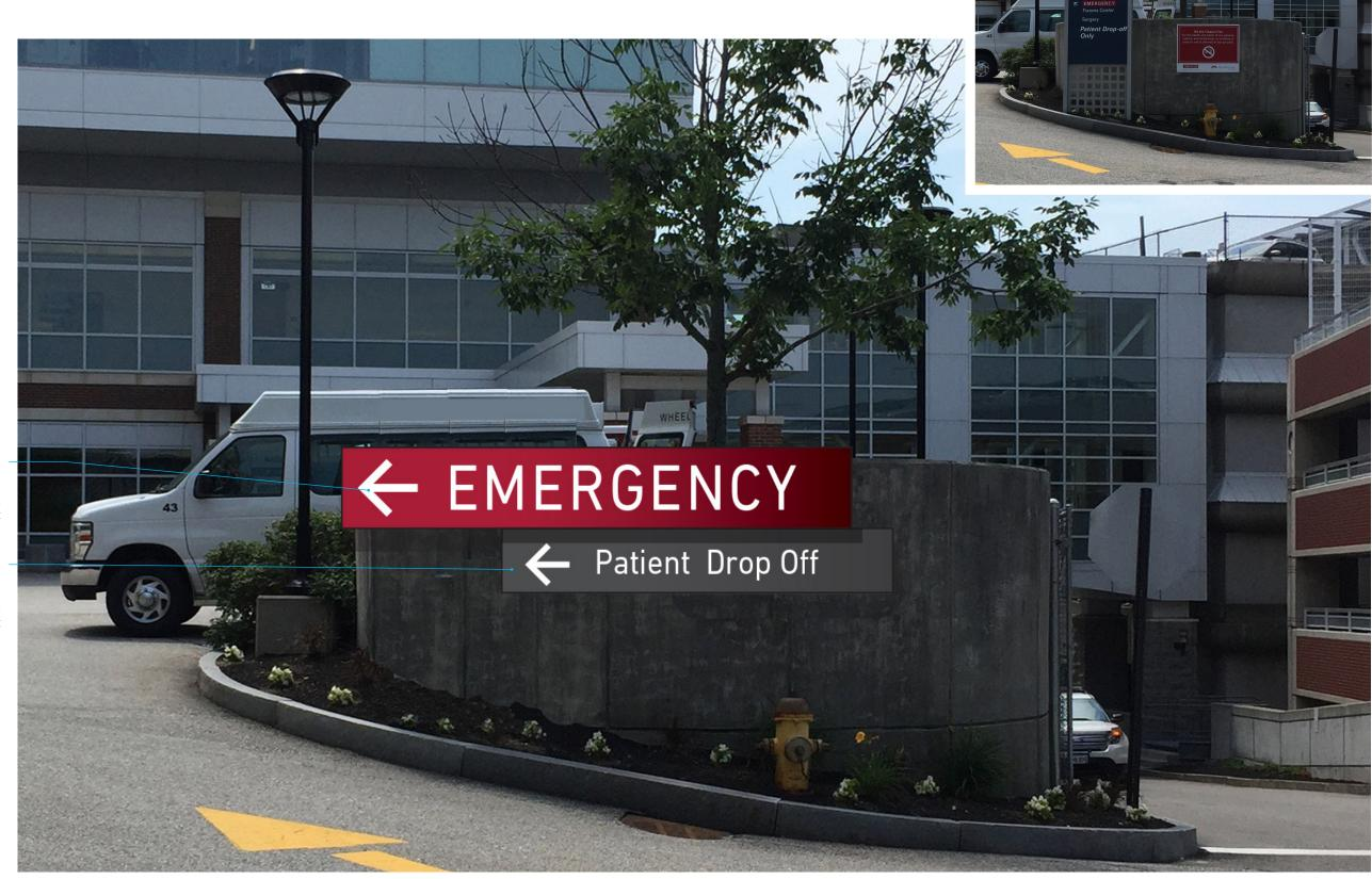
Single sided 16"T x 14'W x 6"D Fabricated painted aluminum sign with internally illuminated push through letters and arrows Roll formed, flush mounted to existing precast
