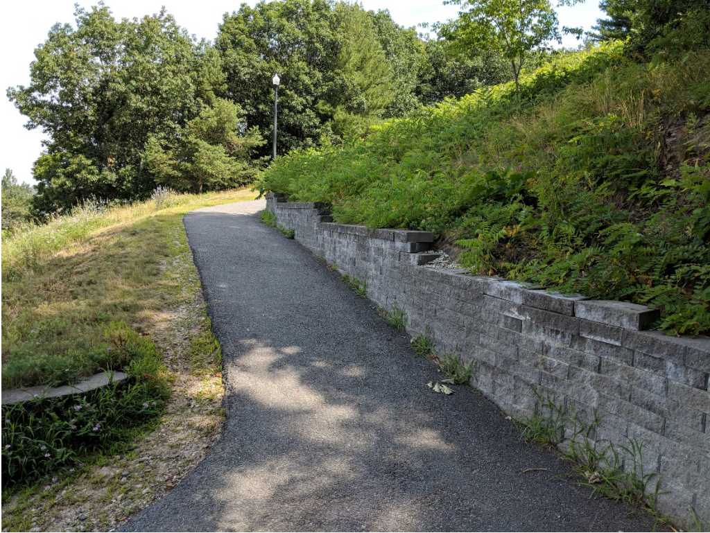
Photo 5: Trail and retaining wall section in good condition
