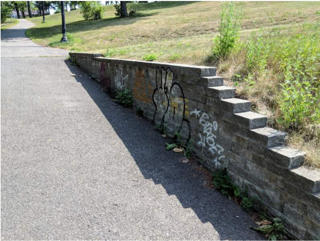
Photo 8: Retaining wall in good condition,
