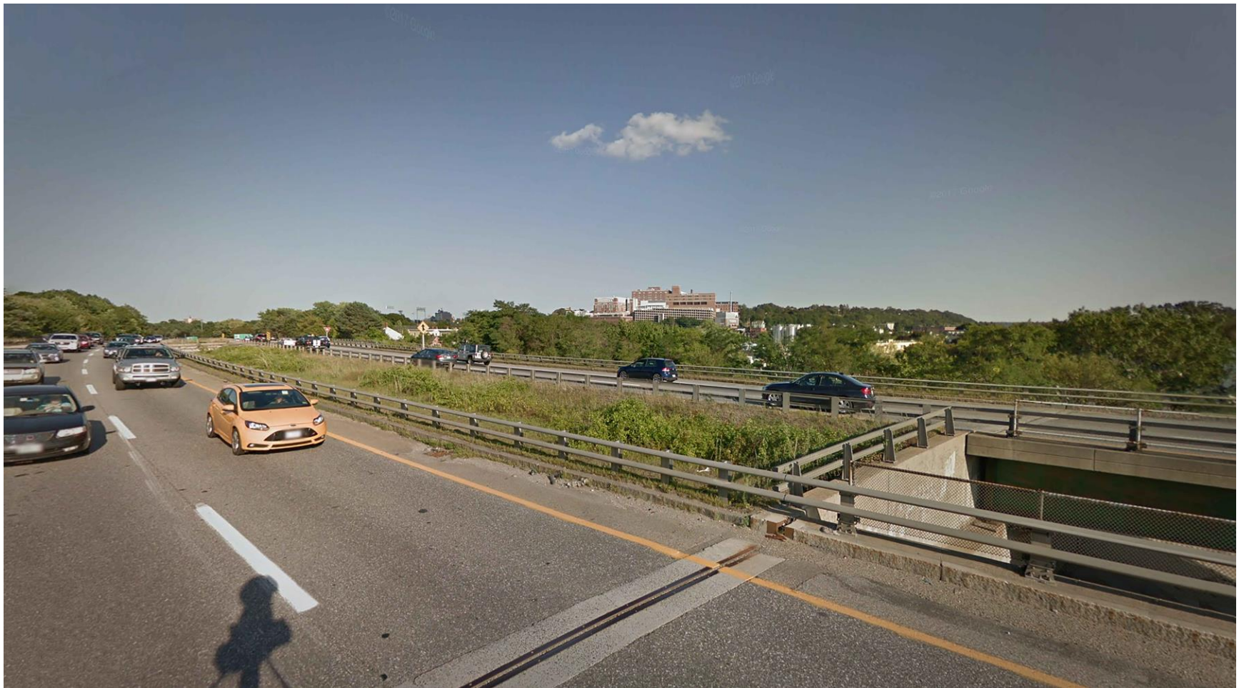
East Tower & Visitor Garage Overbuild As Seen from I-295 Date: 03/23/2018
