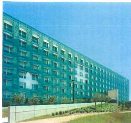
The GSA Field Office in Houston, Texas is a LEED-Certified building that is also bird-friendly. Photo by Timothy Hursley
