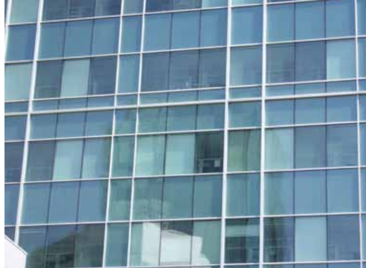
Translucent glass can help balance daylighting and prevent bird collisions
