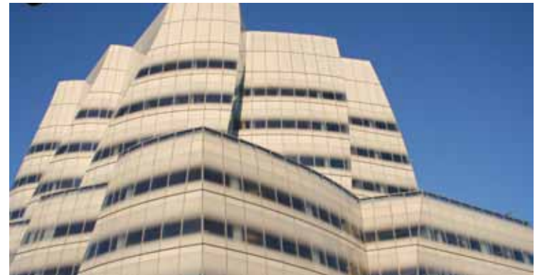
White fritted pattern on glass facade at IAC Offices in New York City
