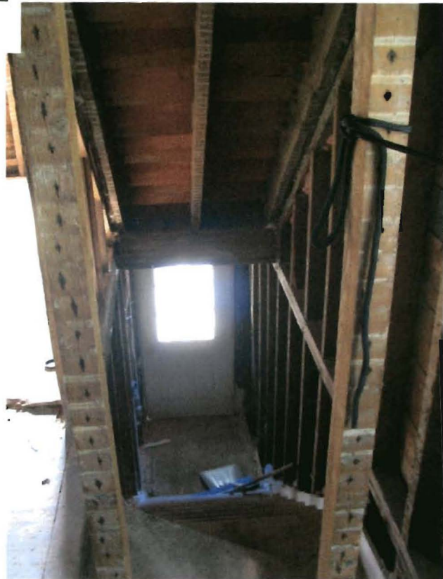
Stairway at front entry
