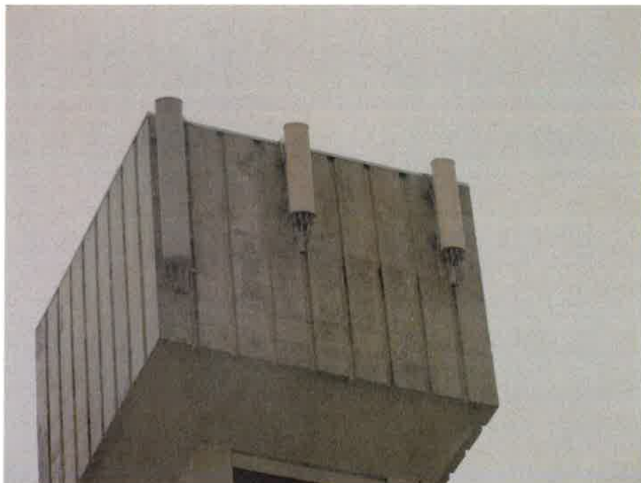
Photo 2: Sample photo illustrating the existing façade-mounted antennas.
