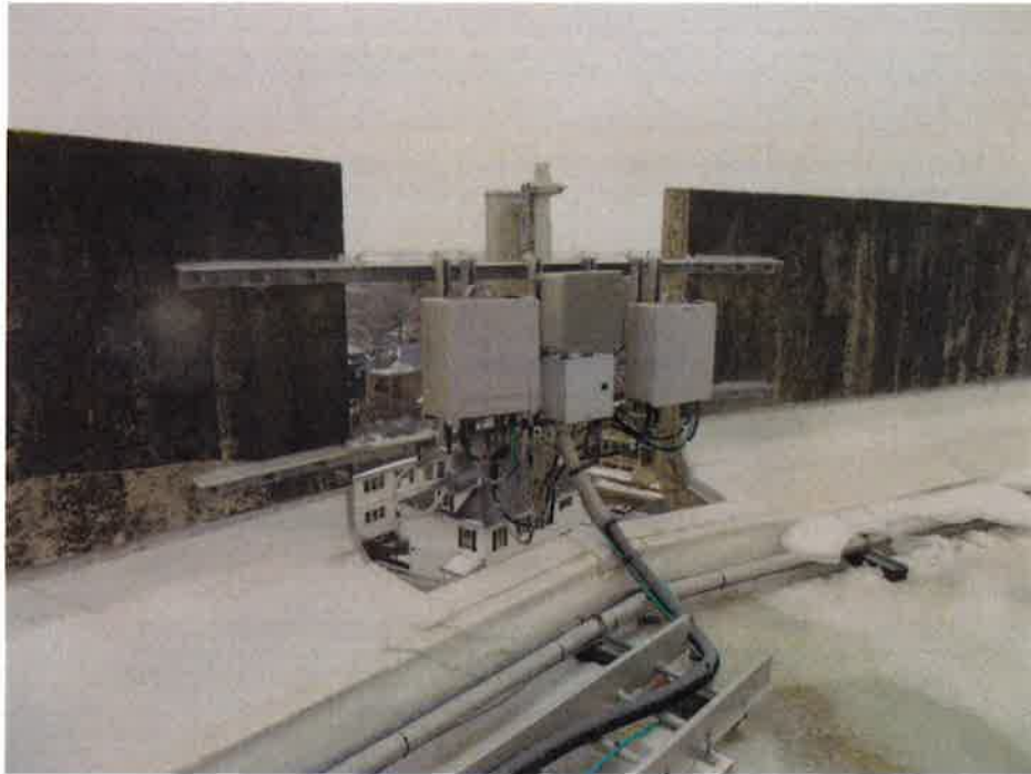
Photo 1: Sample photo illustrating the existing antenna support angles.
