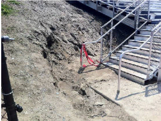
Right Stair Landing Before
