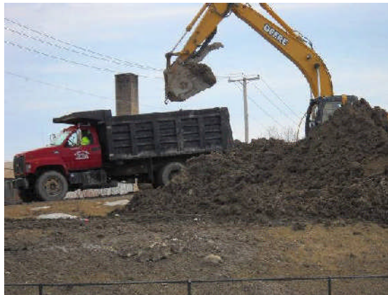
Offsite Material to Replace Unsuitable Soils
