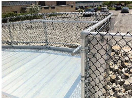
ADA Ramp Handrail Before
