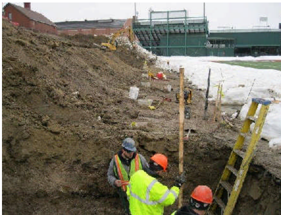
Excavation for Bleacher Footing
