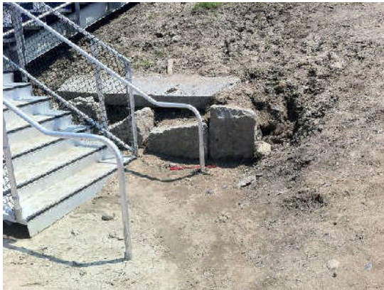
Left Stair Landing Before
