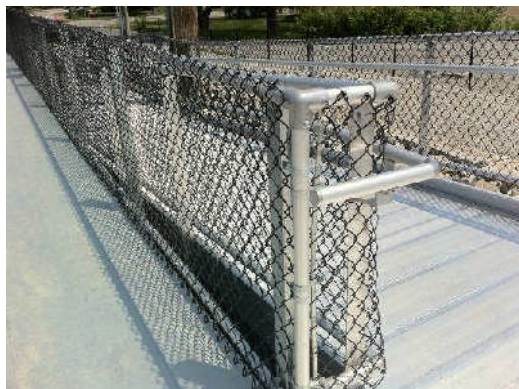
ADA Ramp Handrail Before
