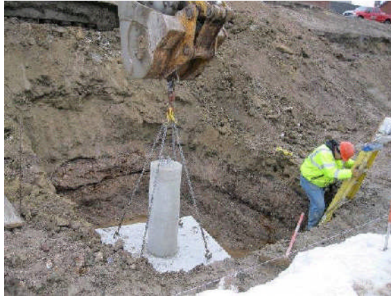
Precast Footing Placed on Subgrade
