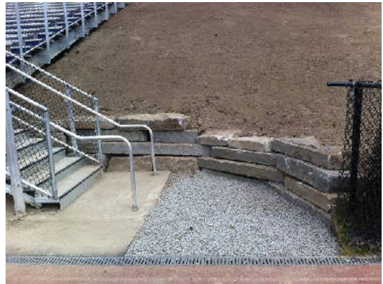
Left Stair Landing After
