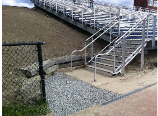
Right Stair Landing After
