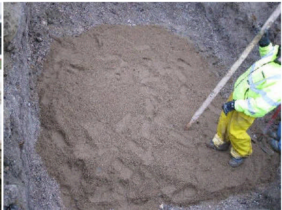
Footing Subgrade with Leveling Sand
