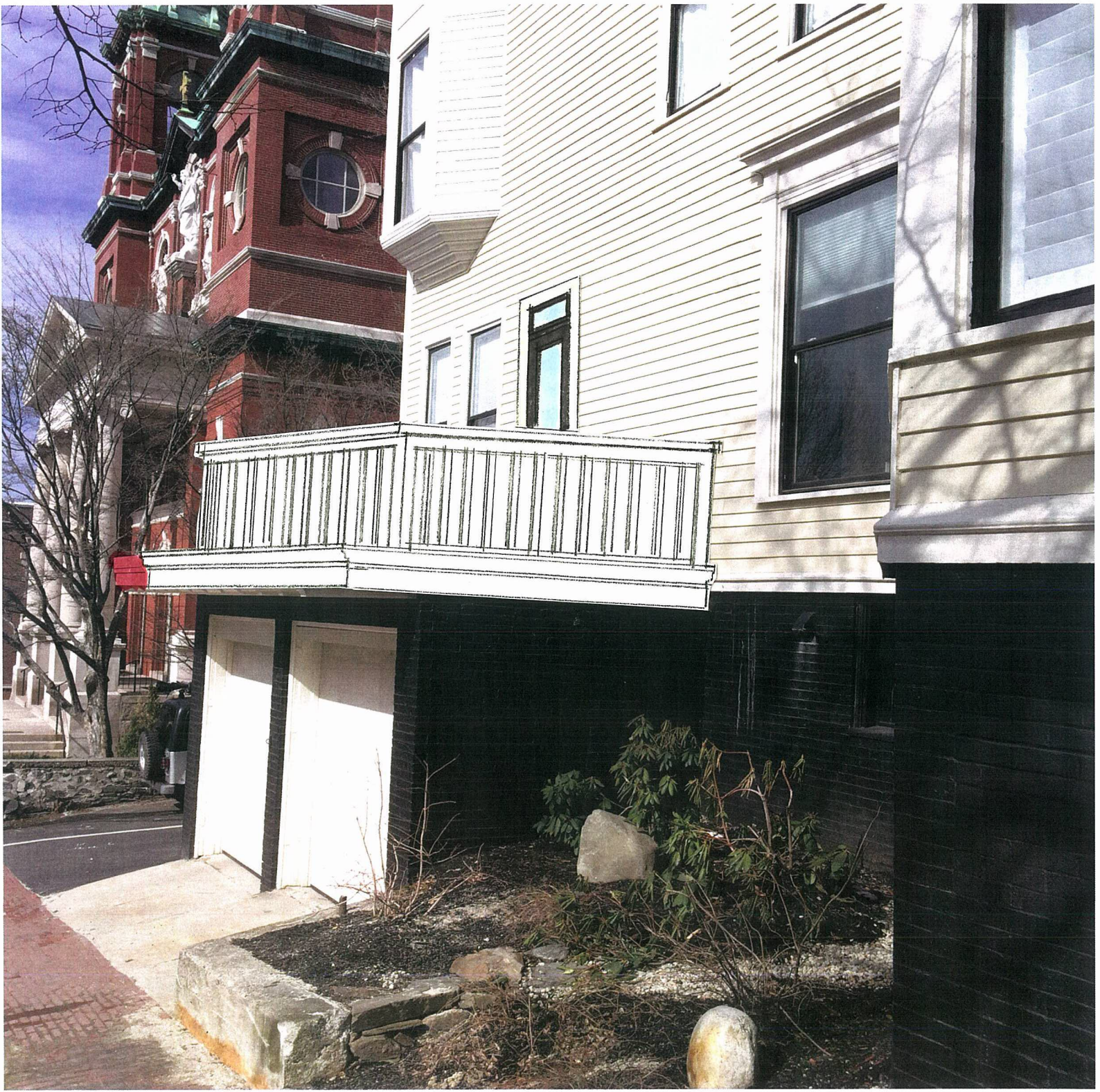
NEW DECK LOOKING SOUTH @ MELLEN ST.
