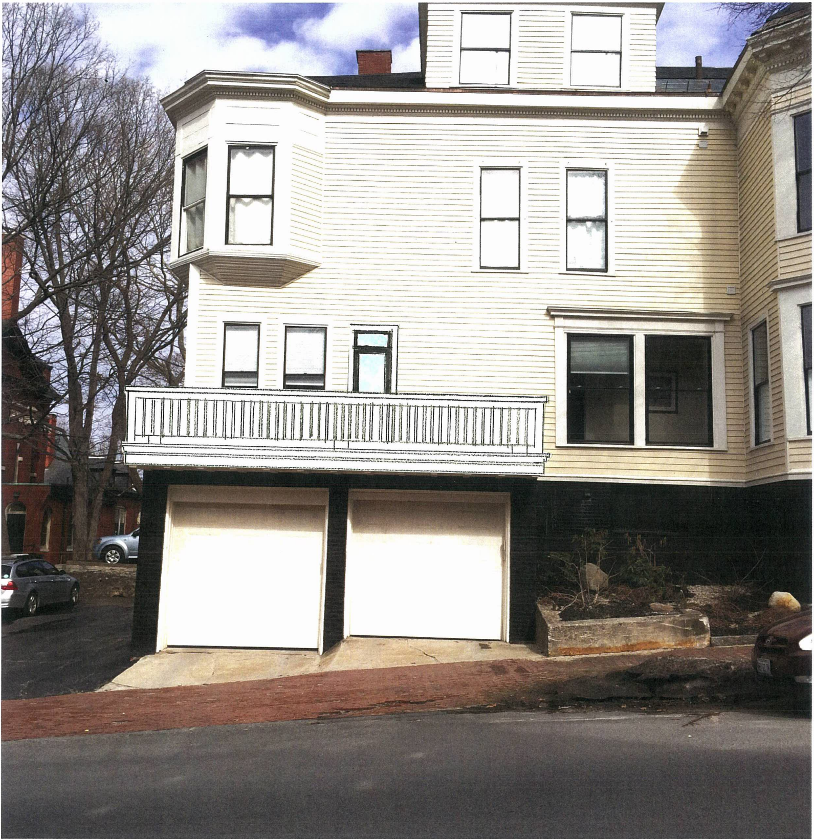
NEW DECK @ MELLEN ST. (WEST) FACADE VIEW
