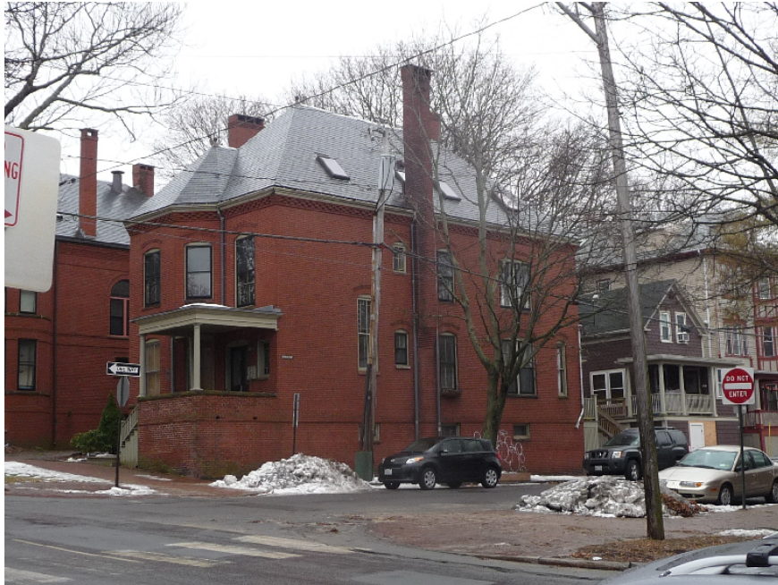
View from State Street
