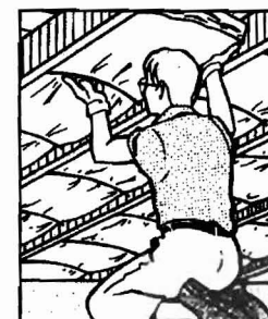
Typical IS Installation
