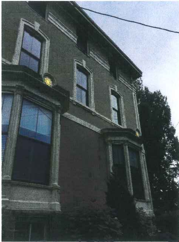
Mellen St. side of the building as it exists today
