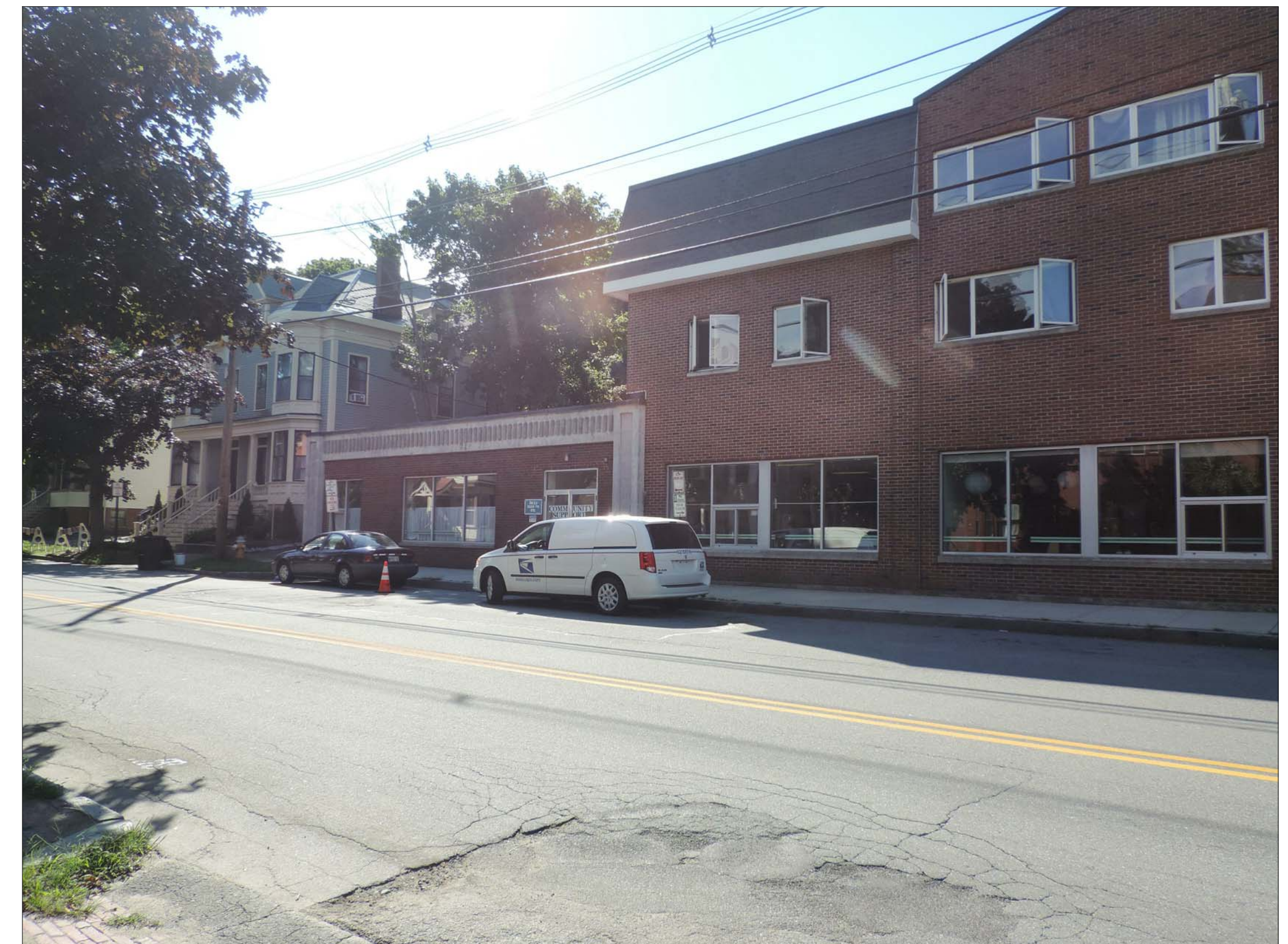
EXISTING BUILDING A FROM CUMBERLAND AVE
