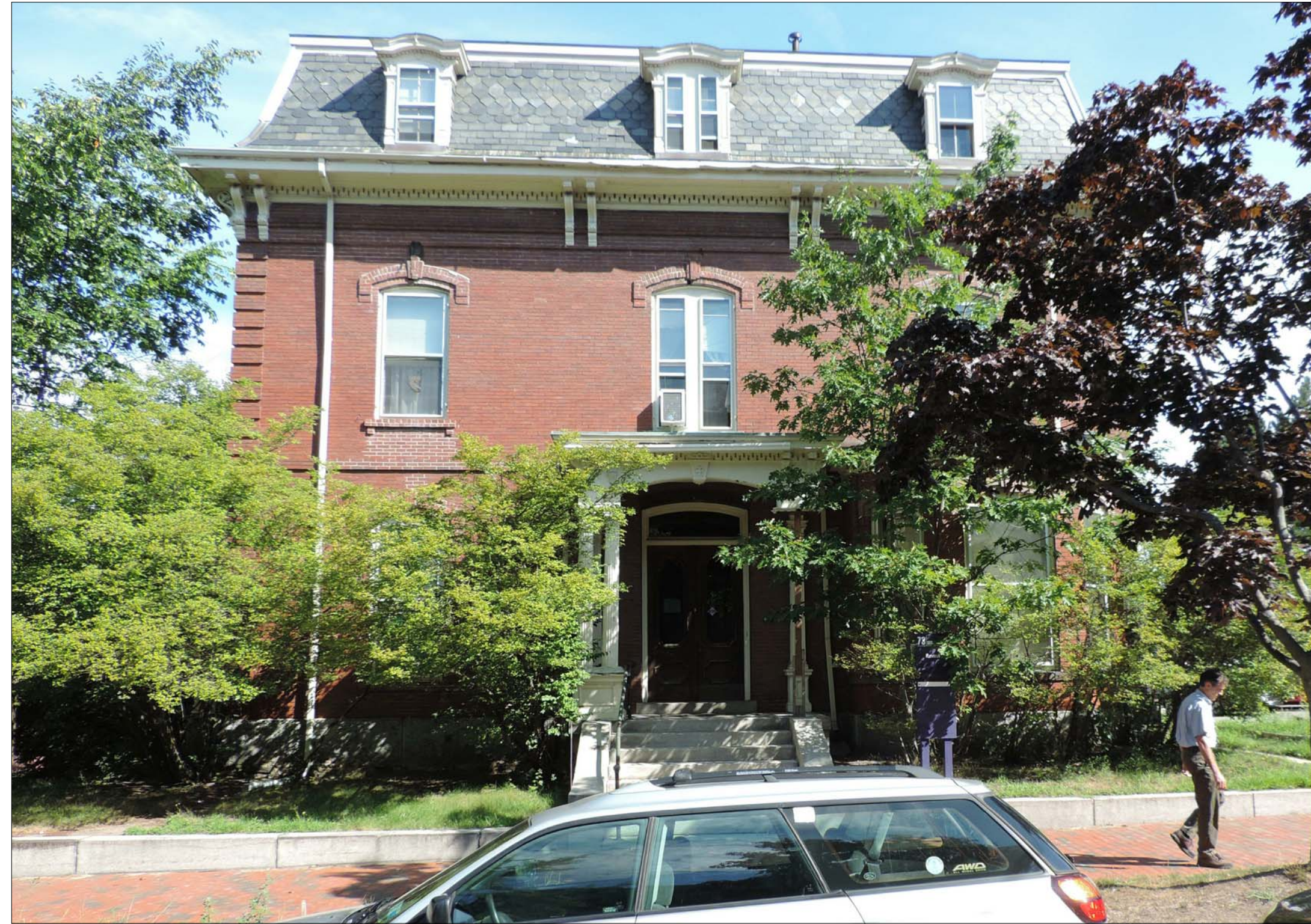
EXISTING BUILDING B FROM DEERING ST
