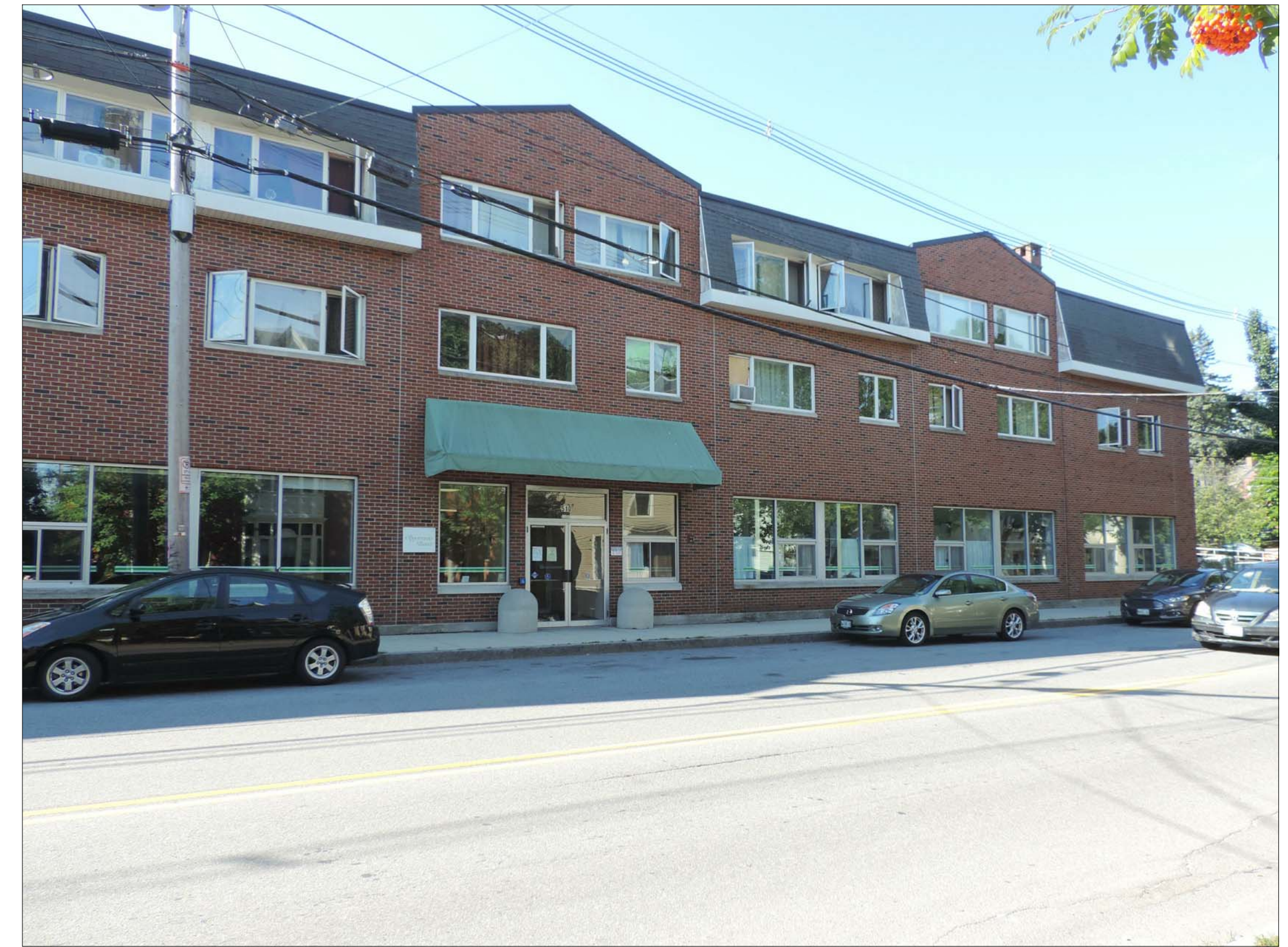
EXISTING BUILDING A FROM CUMBERLAND AVE
