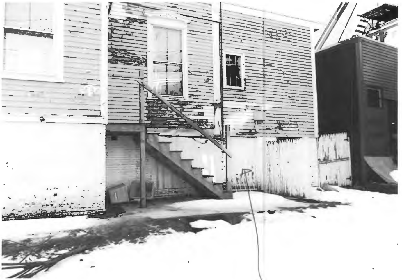
Access Door to basement
