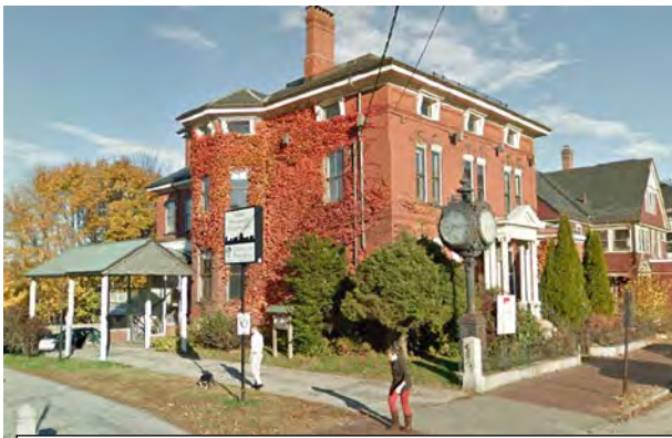
Figure 2: Existing Structure on Congress Street
