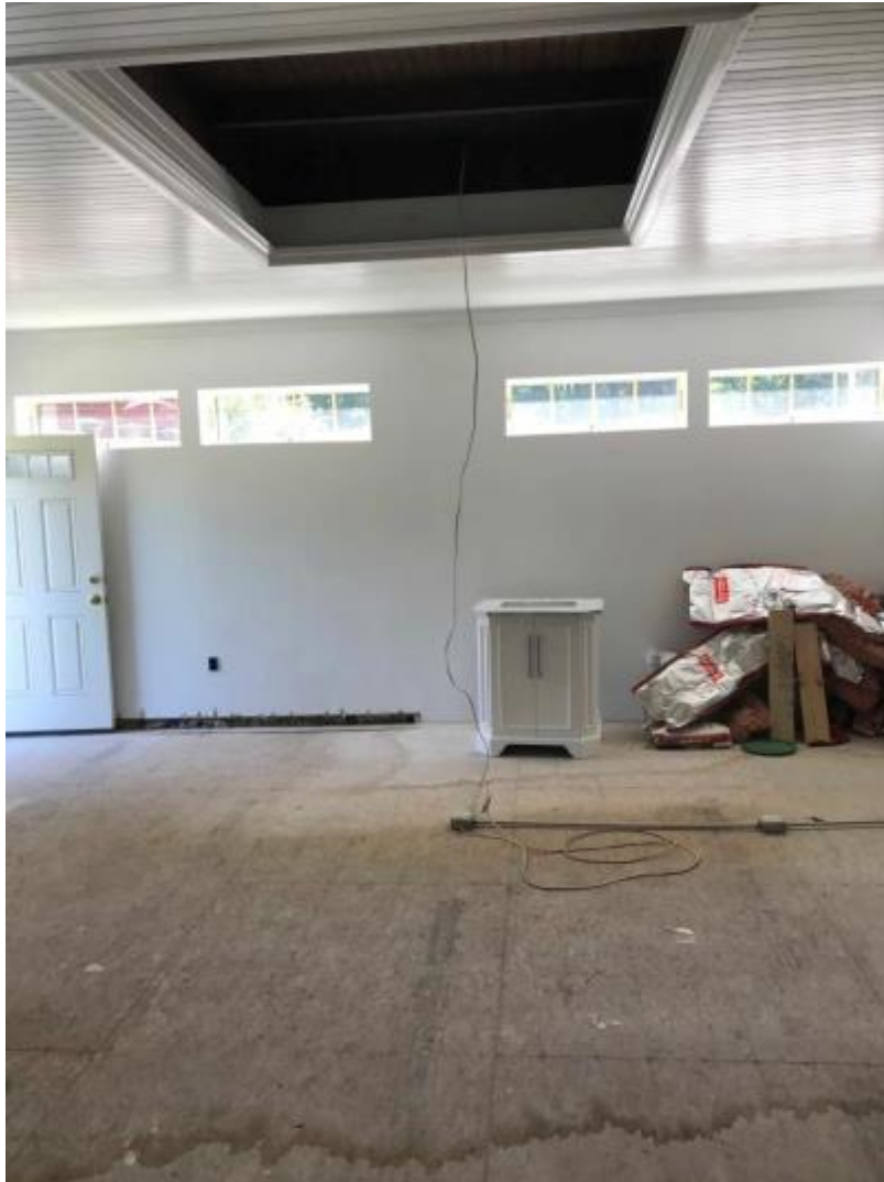
3 IMG_0706 Date Taken: 7/20/2017 Taken By: ANDREW Where garage doors were
