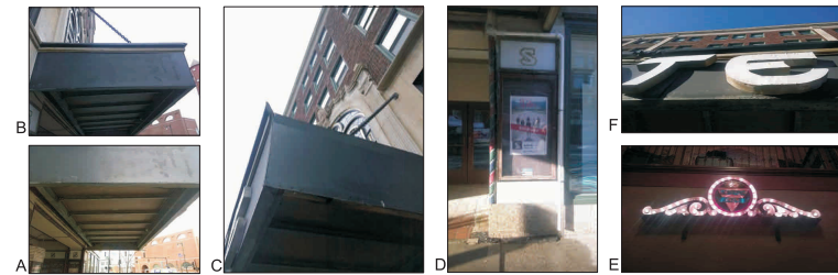
EXISTING CONDITION PHOTOGRAPHS SCALE: NTS
