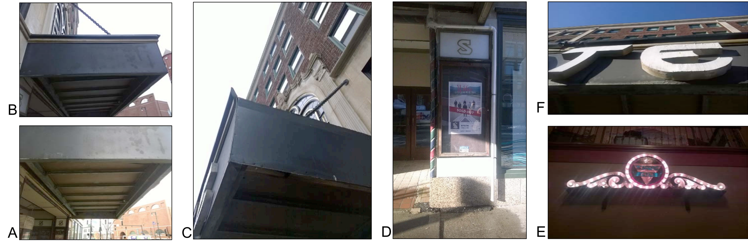
5 EXISTING CONDITION PHOTOGRAPHS SCALE: NTS
