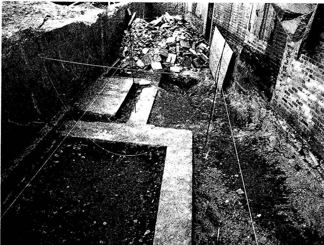
Photo # 2 – Existing first entry foundations and footings (view looking east)
