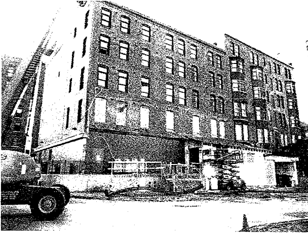
Photo # 1 – Back of building, view looking South
