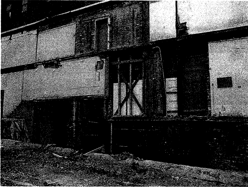
Photo # 1 – Elevation at back wall (view looking South at grid F, near grid 6)
