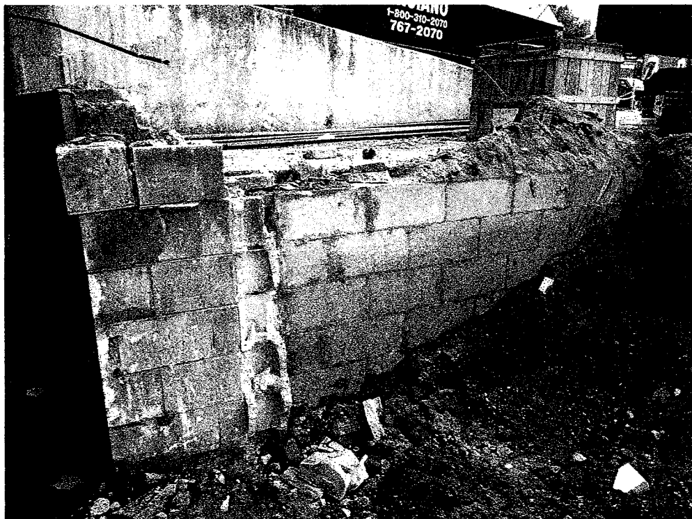
Photo # 4 - Existing ungrouted 8" CMU foundation at grid 4.8 (rear entry)
