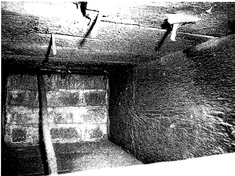
Photo # 2 – Wood framing below existing second-floor bay window at grid F/4.8 mortared into existing brick.
