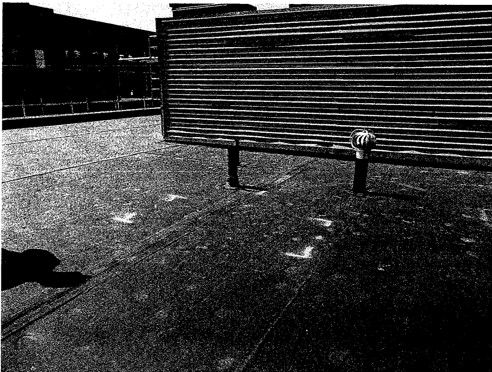
Photo # 2 – Revised relocation of rooftop HVAC ( shown by yellow marking on roof) located over column
