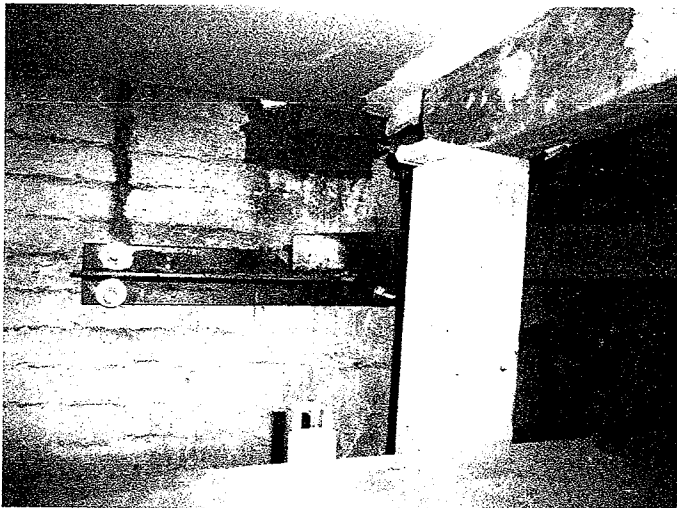
Photo # 9 - Steel brace at Grid A/2.9 foundation wall has been installed.
