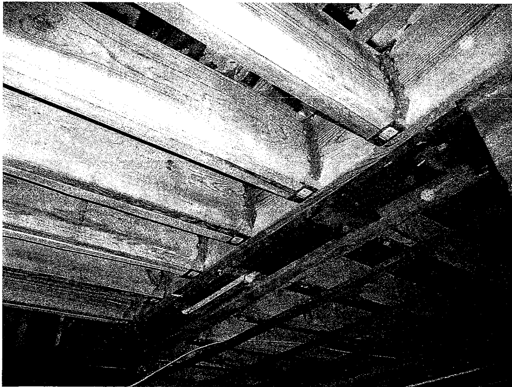
Photo # 2 – Double joists at 1 st Floor Grid a.5/9.5. Header must be bolted to existing beam.
