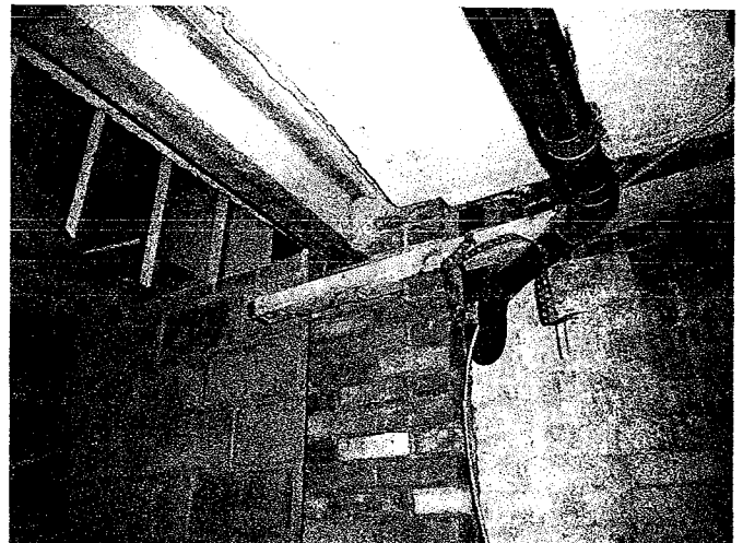
Photo # 10 - Rebuilt Bearing @ Grid F.3/2.5 (Looking NE)
