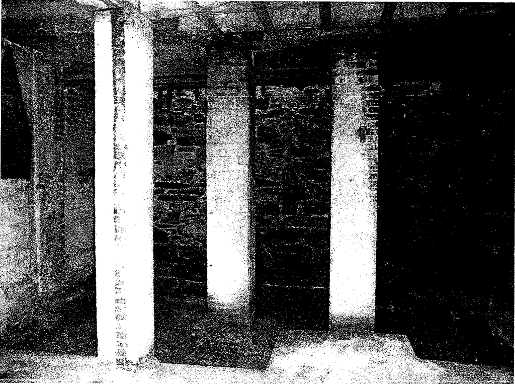
Photo # 5 – Existing brick column and footing in basement at grid A./8 (shown at center).
