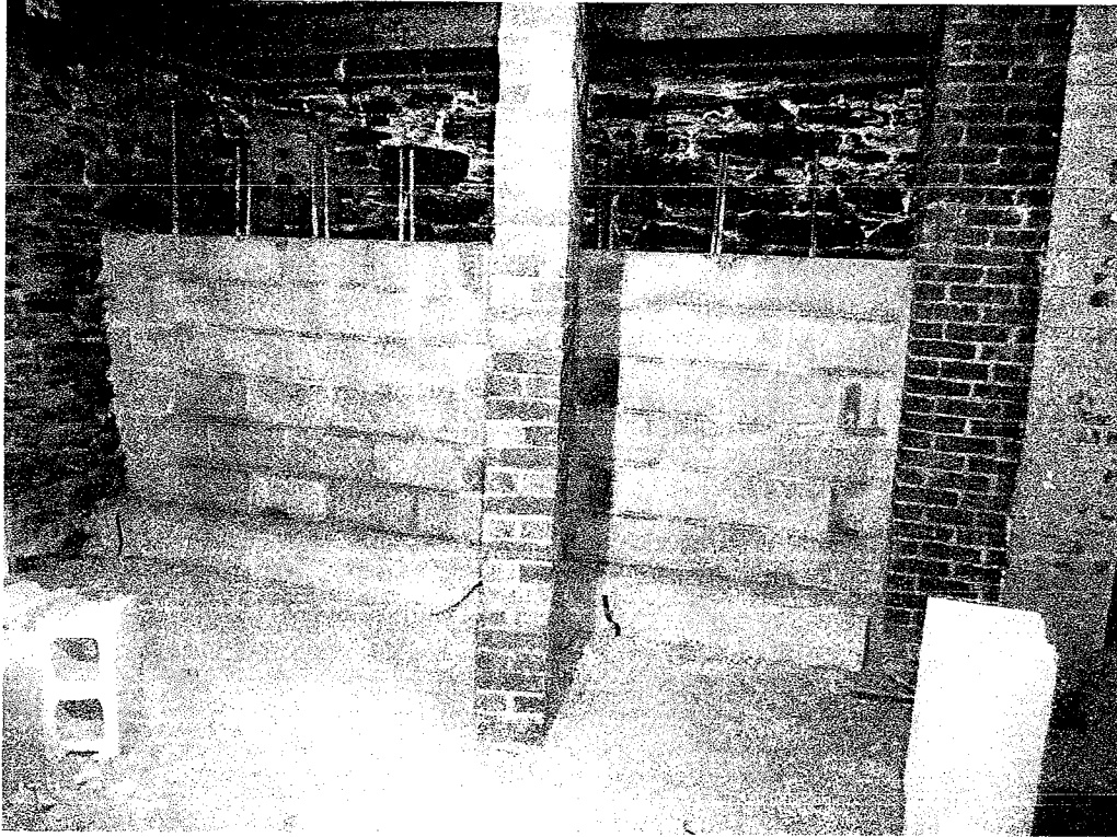
Photo # 1 – Four foot tall 8” CMU at basement grid A/8 to A/10
