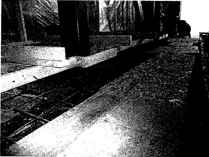
Photo # 4- Cantilevered formwork to accommodate concrete step for brick shelf.
