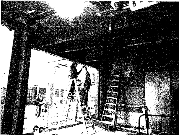
Photo # 6 – Installation of steel beams above main entrance.
