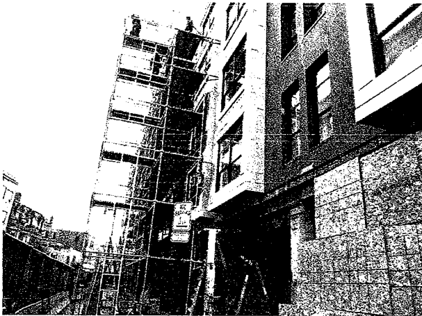
Photo # 2- Scaffolding being removed in front of building
