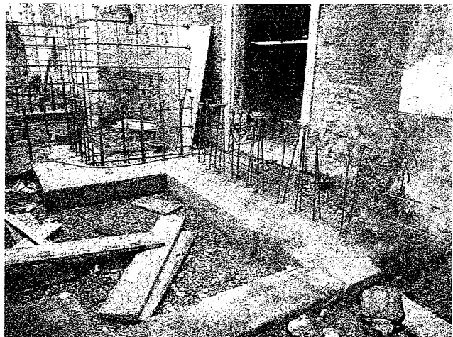
Photo # 6 – Reinf. @ rear retaining wall fig. (Grid F.4/5.2)
