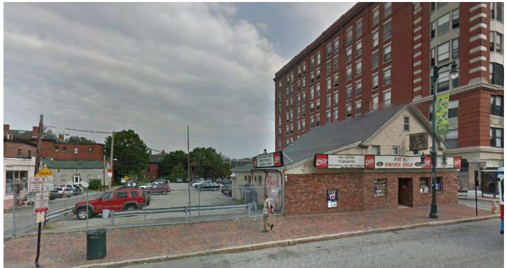
Figure 1- Existing Site from Congress Street
