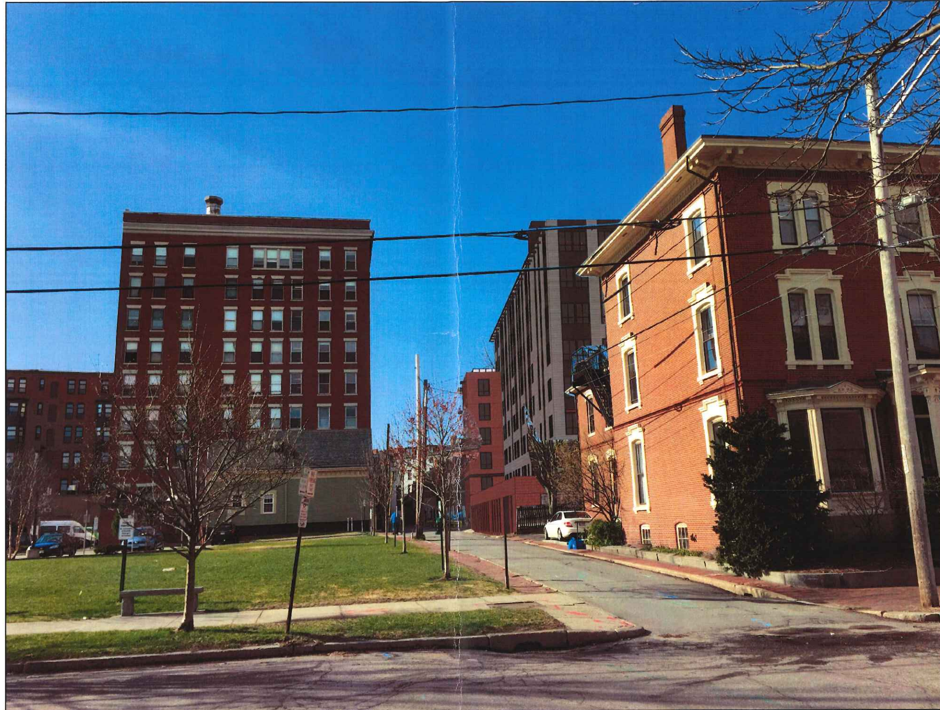
VIEW LOOKING SOUTH FROM DEERING STREET
