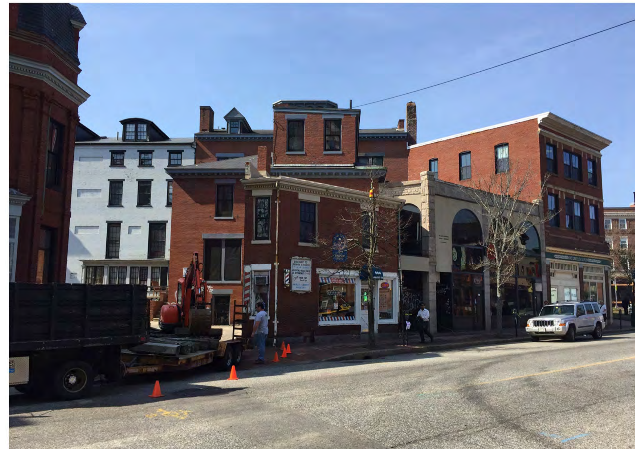
VIEW LOOKING NORTHEAST ON CONGRESS ST
