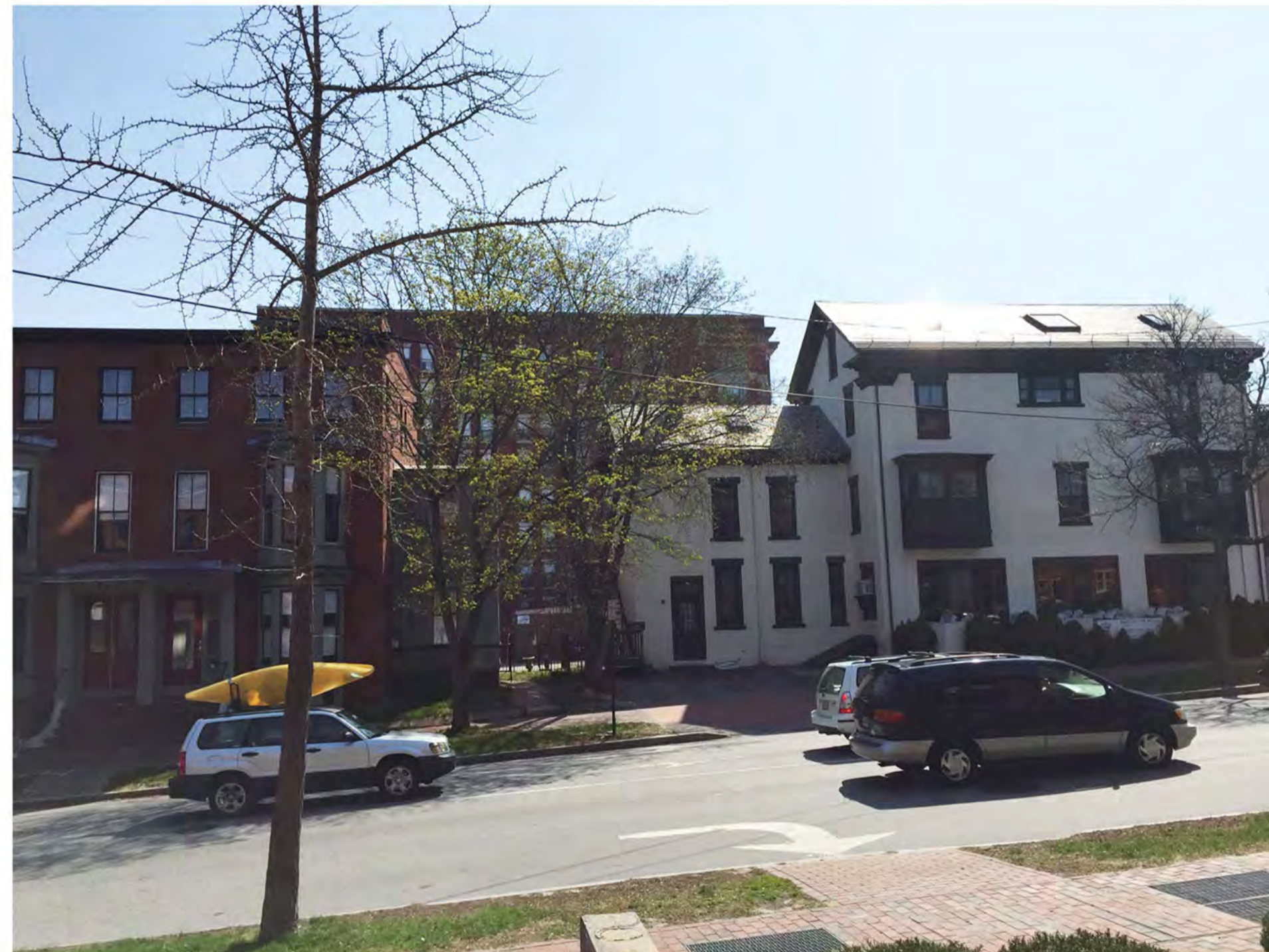
VIEW LOOKING EAST FROM STATE STREET
