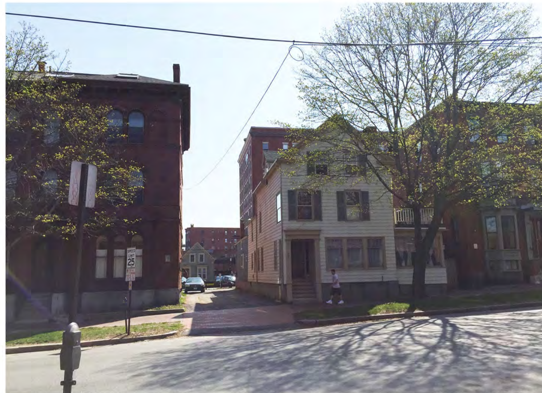
VIEW LOOKING EAST FROM STATE ST
