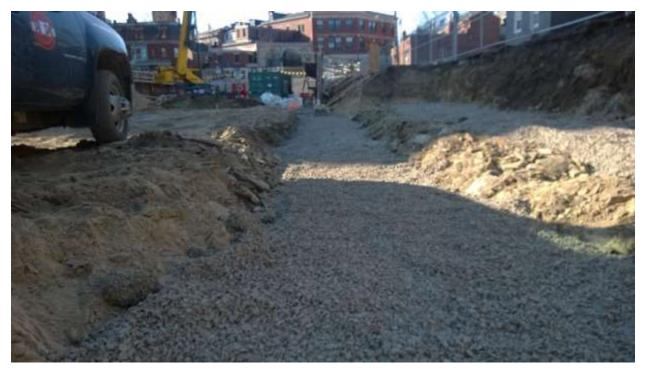
Photograph 2 – Crushed stone subgrade on building line 7 south of line F; Date 05 April 2016
