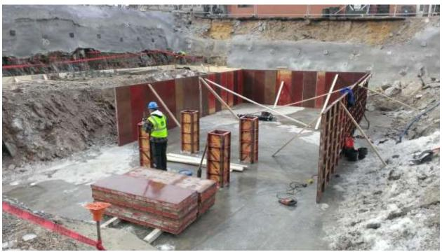
Figure 4 - Mass concrete footing subgrade in area of building line M.9 to P.3. Photograph date: 04 March 2016
