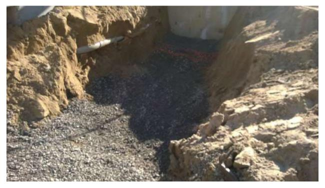
Photograph 6 - Crushed stone over bedrock on building line C.2 between lines 1.2 and 2.3. Date: 21 April 2016
