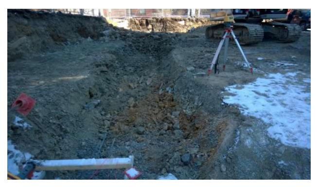
Photograph 1 – Exposed subgrade on building lines 7 and 8 from line E to F prior to placing crushed stone. Date: 05 April 2016
