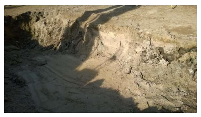
Photograph 5 – Storm drain trench backfill at foundation subgrade level on building line 2.3 between lines C.2 and C.9. Date: 20 April 2016.
