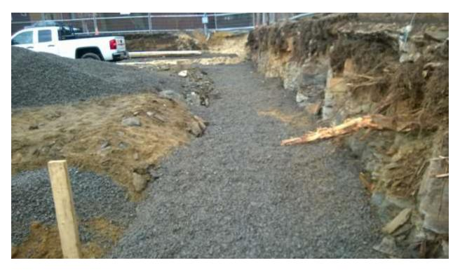
Photograph 3 – Crushed stone over bedrock on west part of building line A. Date: 06 April 2016
