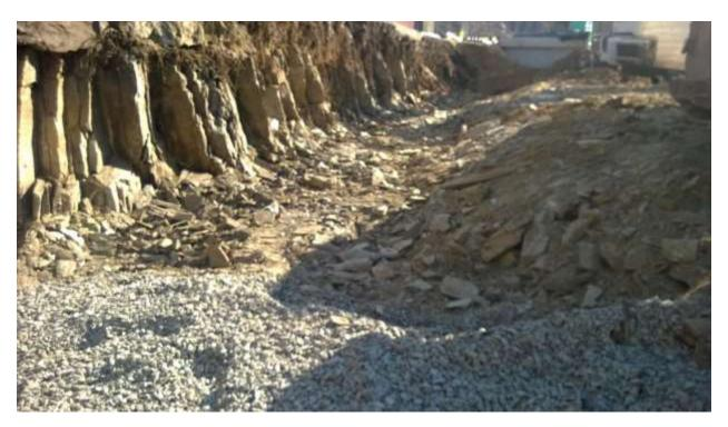
Photograph 4 – Exposed bedrock in east part of the building line A prior to placing crushed stone. Date: 06 April 2016
