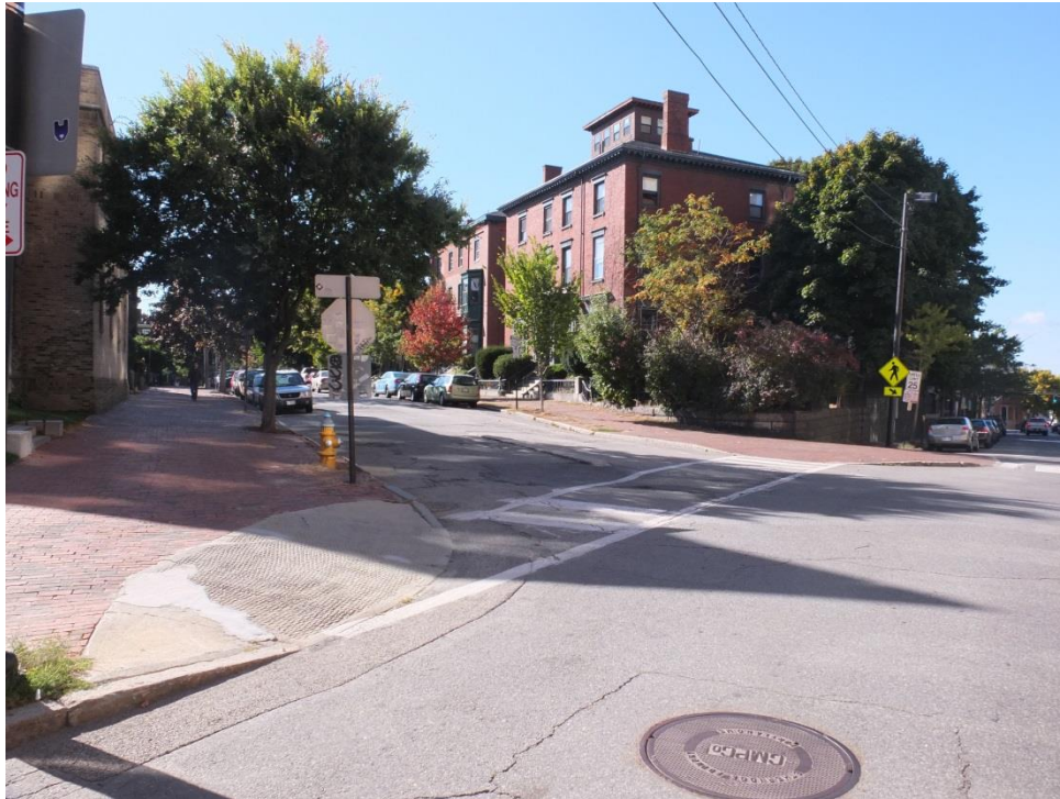
Existing view of Deering Street, facing north from High Street.
