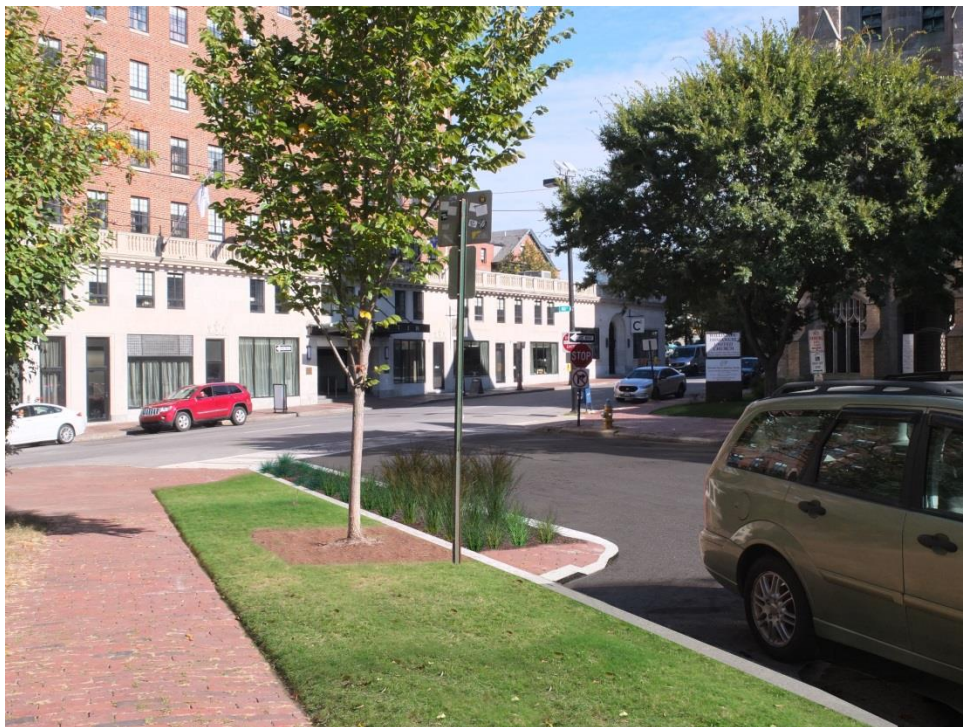
View of Deering Street showing the proposed streetscape and storm water treatment.
