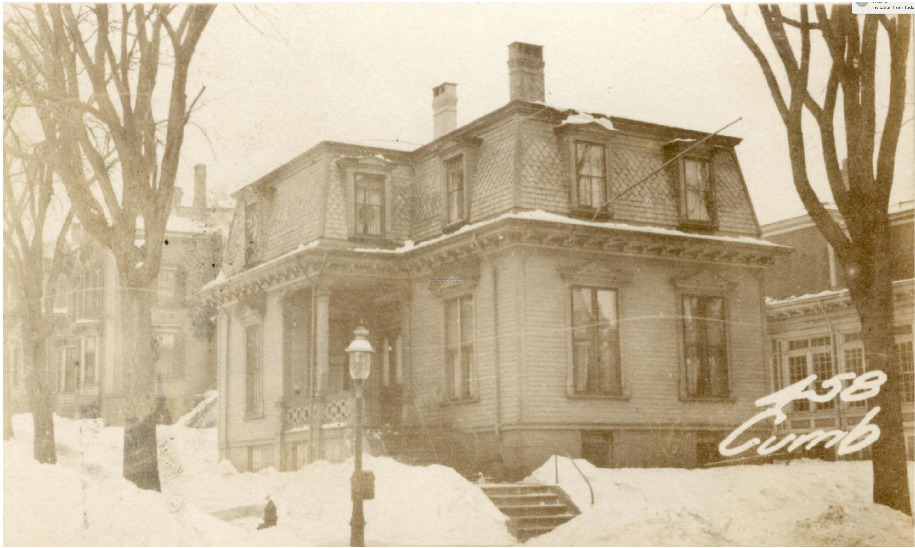
CITY OF PORTLAND TAX RECORDS PHOTO
