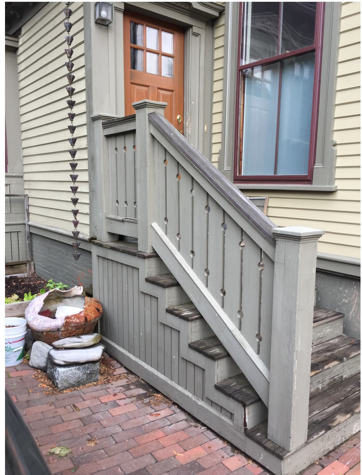
EXISTING STAIR AT BACK ENTRY
