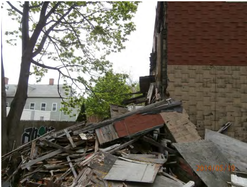
11. Image showing wood debris at the Site.
