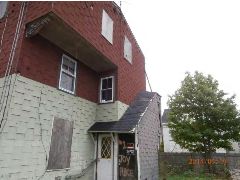
2. Image showing the Site residential building, view facing east.
