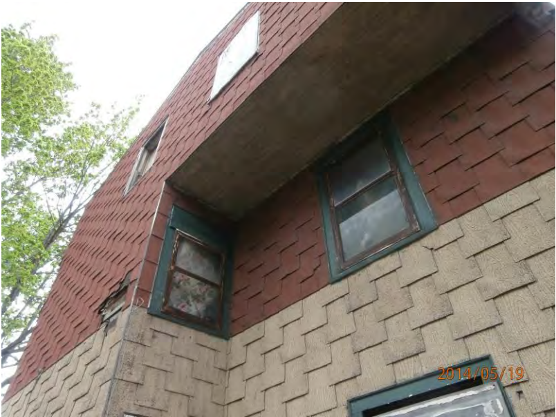
3. Image showing the Site residential building.
