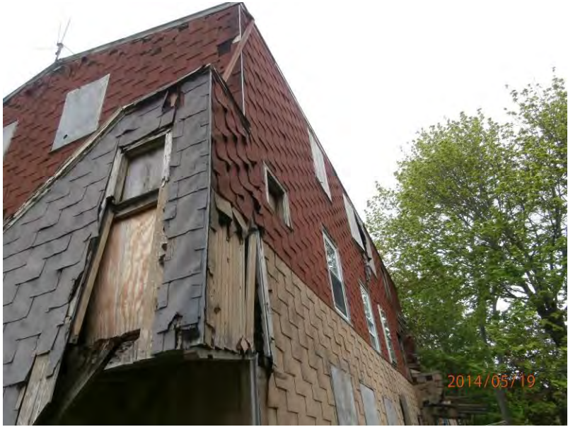
4. Image showing the Site residential building, view facing west.
