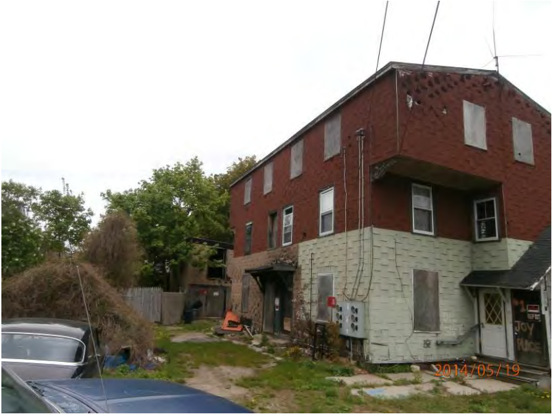
1. Image showing the Site residential building, view facing north.
